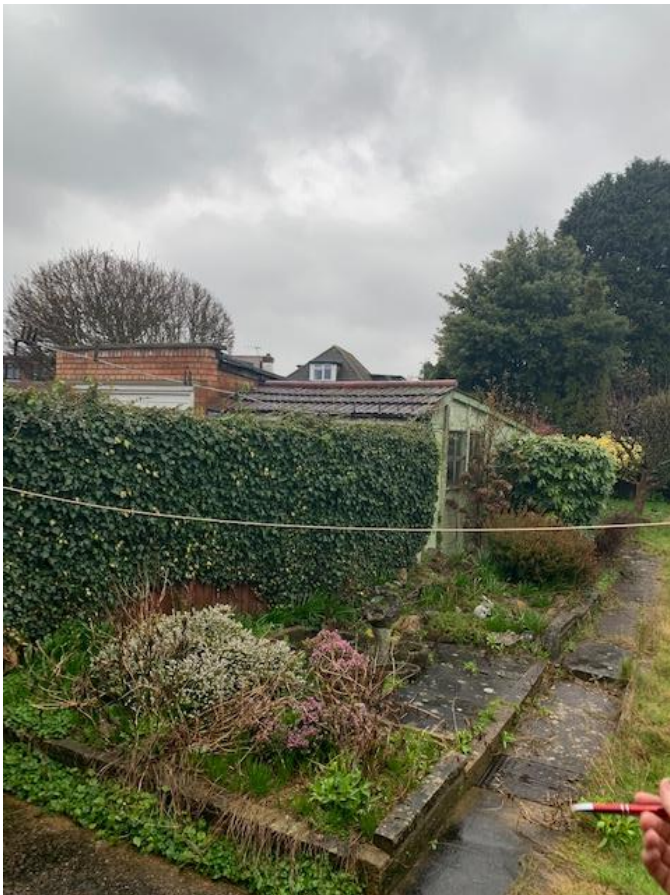
Photograph 03 – existing detached garage
