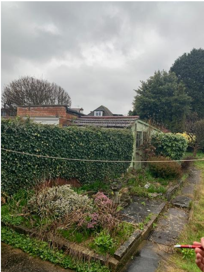
Photograph 03 – existing detached garage
