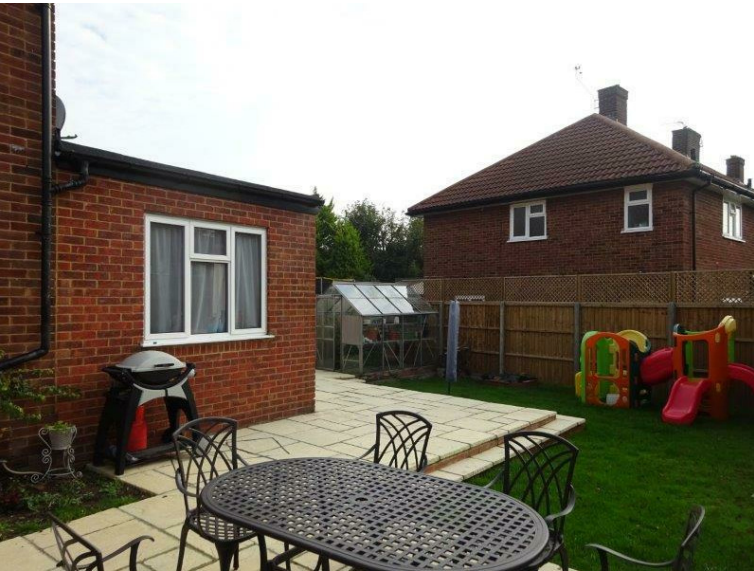
400-10 View Of Extension to 29 Seymour Gdns & Terrace
