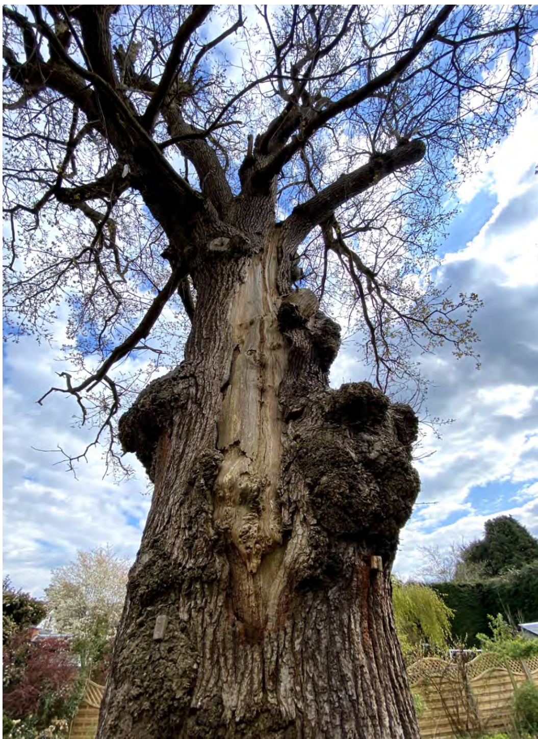
Photographic plate showing the stem wounding, delamination of bark and cracking which extends from the branch unions down to 2-2.5m above ground level.
