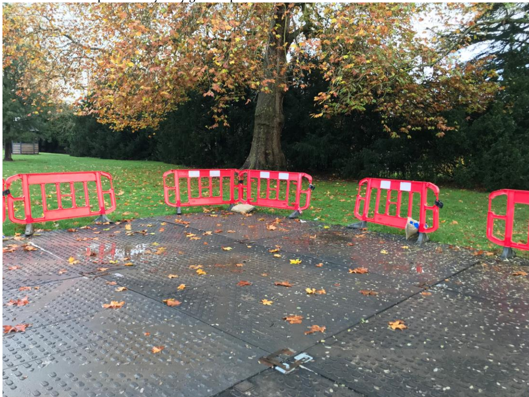
Photo 2. An example of heavy duty ground protection.
