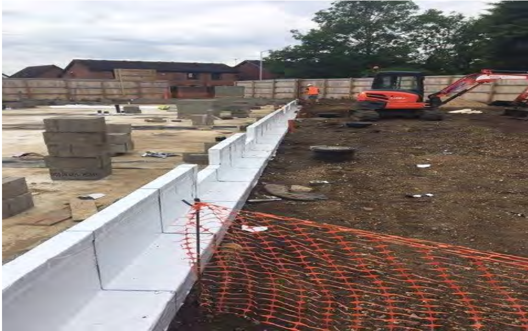
JUTA GP1 gas membrane to infill area
