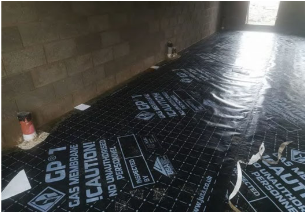
JUTA GP1 Gas membrane with GRSAM repairs
