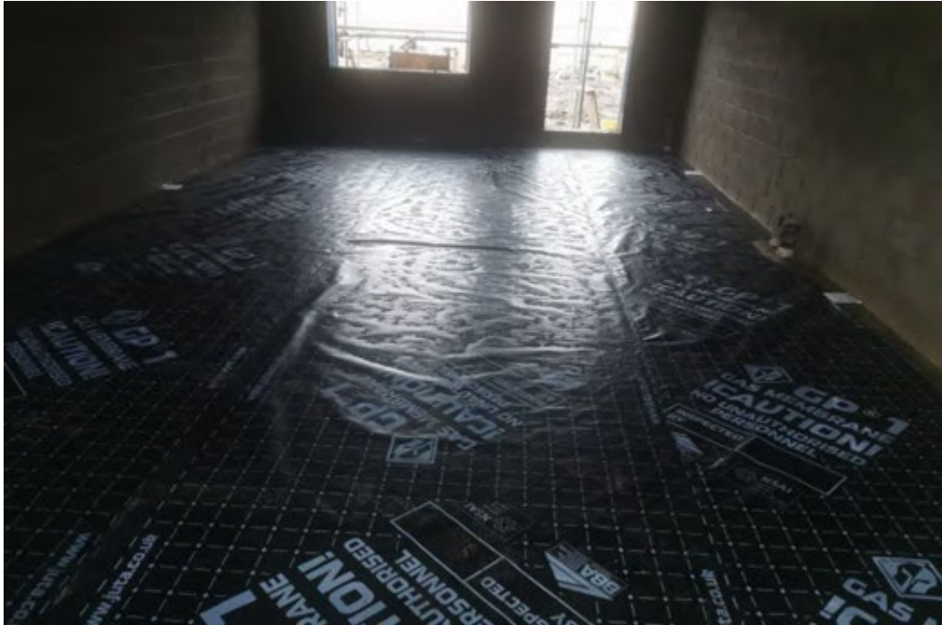
JUTA GP1 with JUTA GRSAM repairs to internal walls membrane
