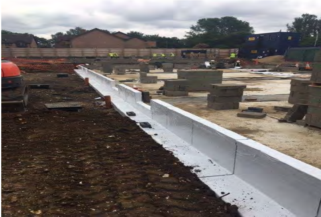
JUTA GP1 gas membrane with JUTA GRSAM detailing work
