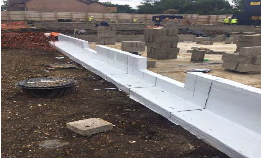
JUTA GRSAM system to perimeter walls
