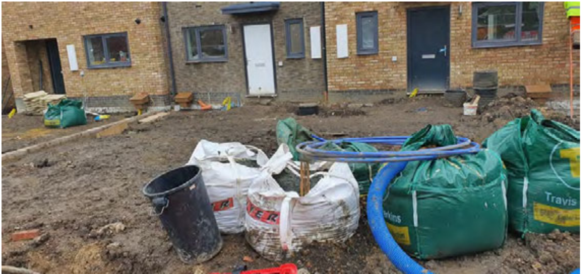
Photograph 29: View of Plots 6-10 prior to the placement of hardstanding.
