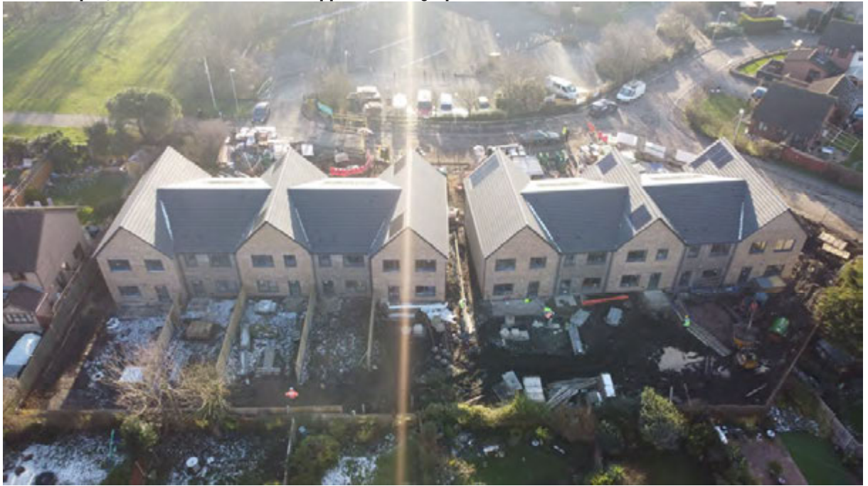
Photograph 5: General site view.
