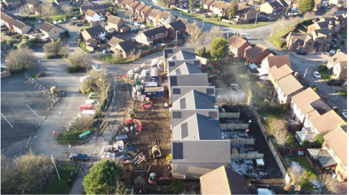
Photograph 7: General site view.
