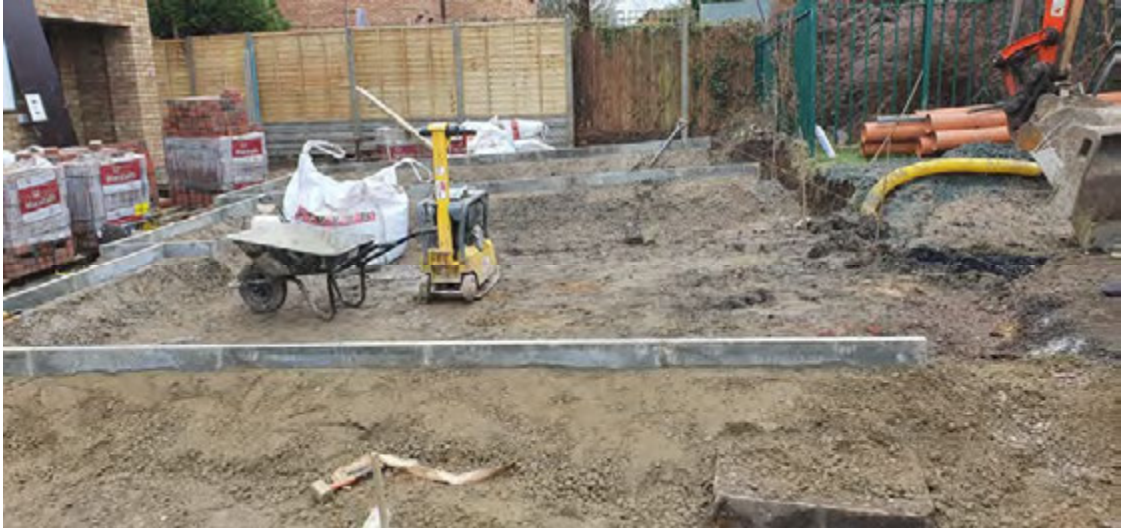
Photograph 26: View of Plots 6-10 prior to the placement of hardstanding.
