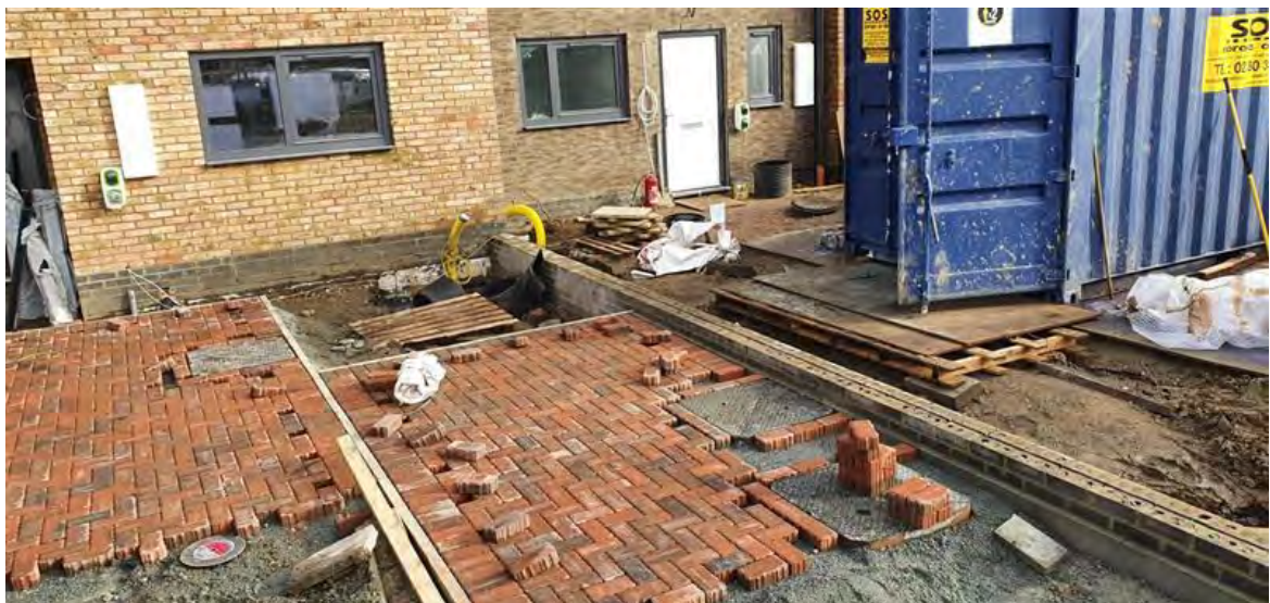
Photograph 19: View of the placement of hardstanding within Plots 1-5.
