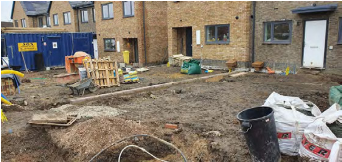
Photograph 27: View of Plots 6-10 prior to the placement of hardstanding.
