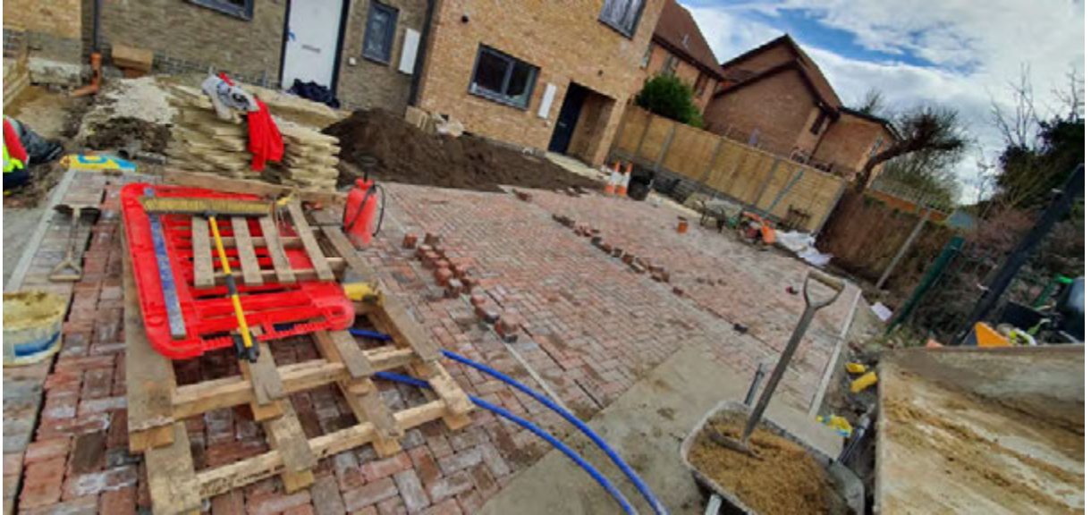
Photograph 35: View of the placement of hardstanding within the front of the properties.
