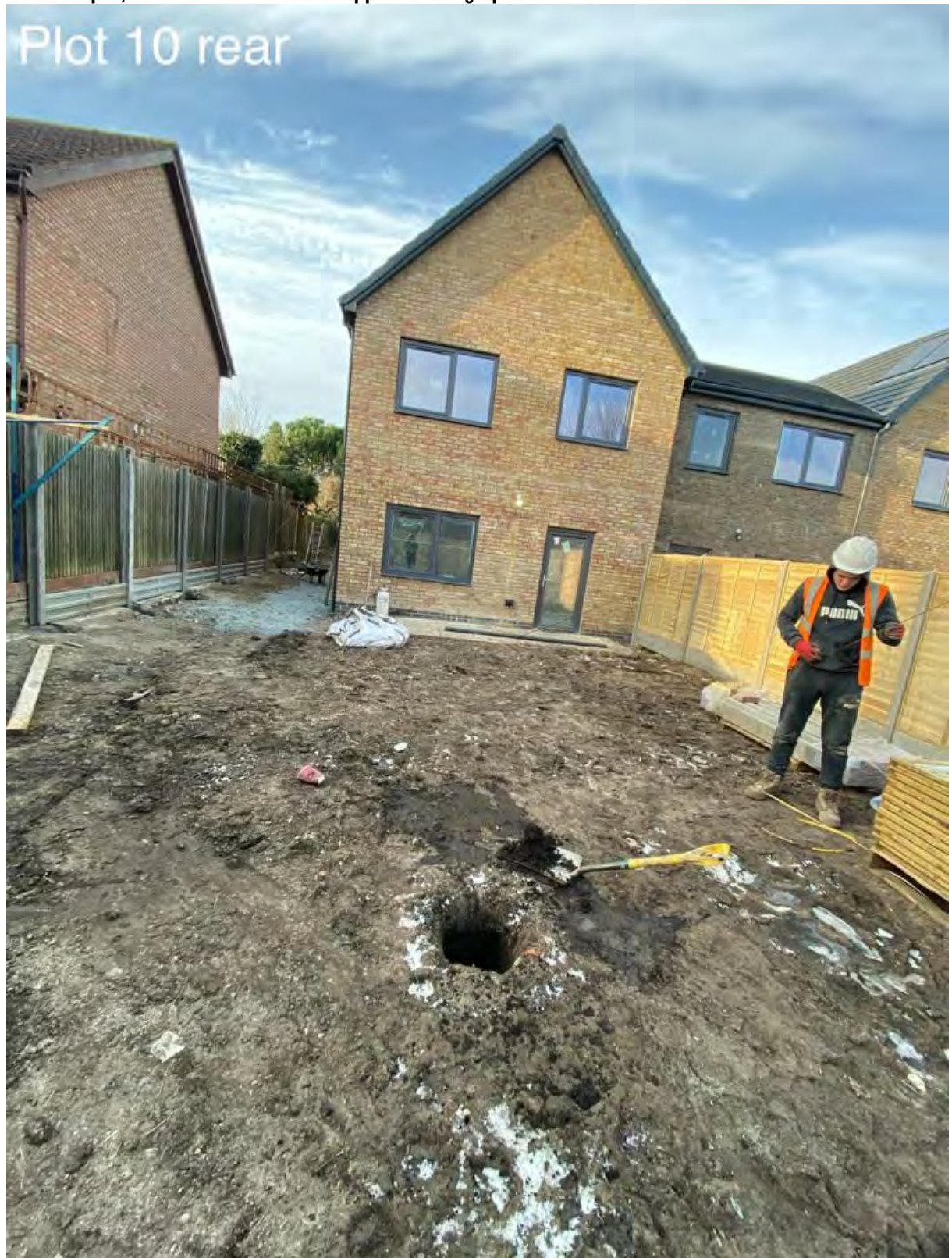
Photograph 12: Verification pit advanced within rear garden of Plot 10.
