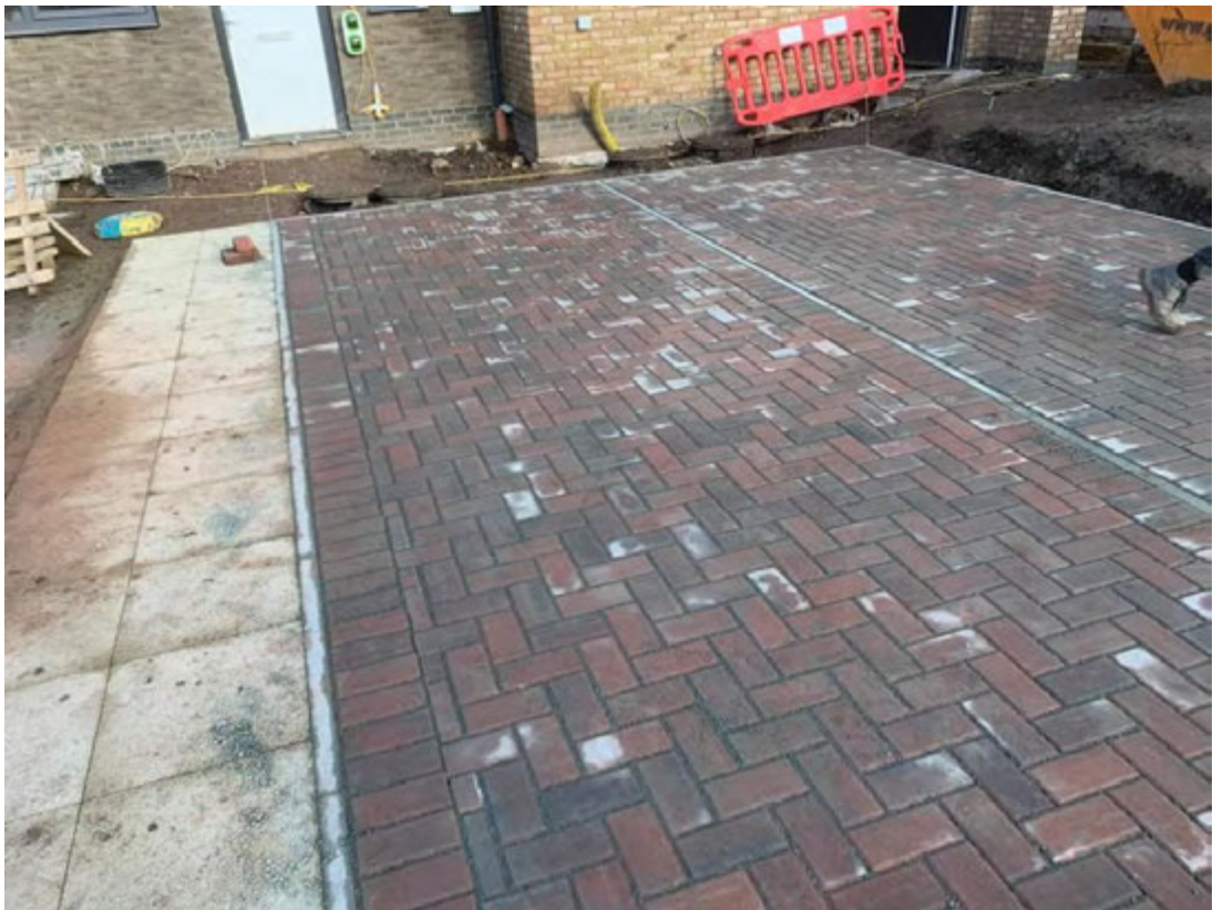
Photograph 23: View of the placement of hardstanding within Plots 1-5.
