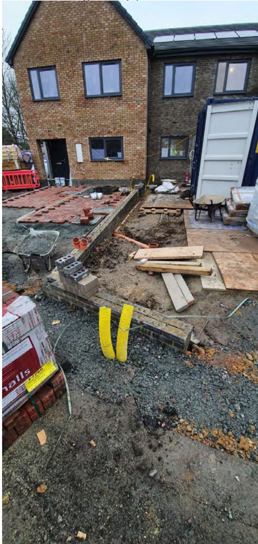
Photograph 21: View of the placement of hardstanding within Plots 1-10.
