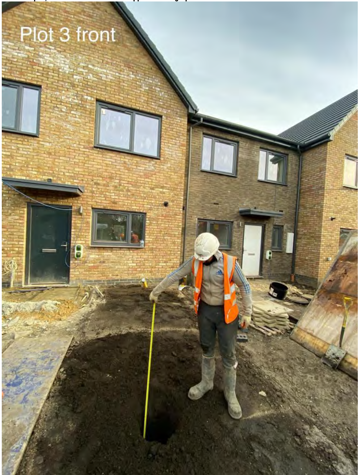
Photograph 9: Verification pit advanced within front garden of Plot 3.
