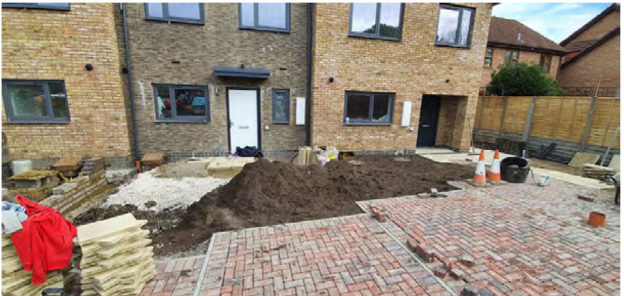
Photograph 36: View of the placement of hardstanding within the front of the properties.
