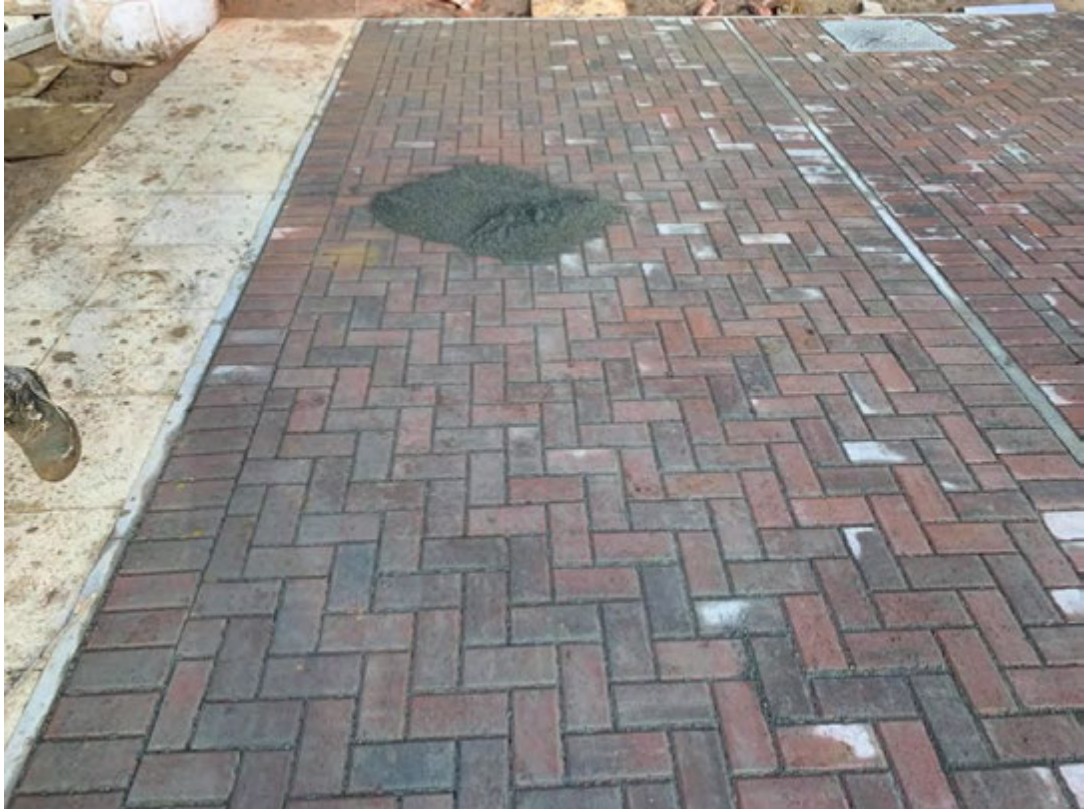
Photograph 22: View of the placement of hardstanding within Plots 1-5.
