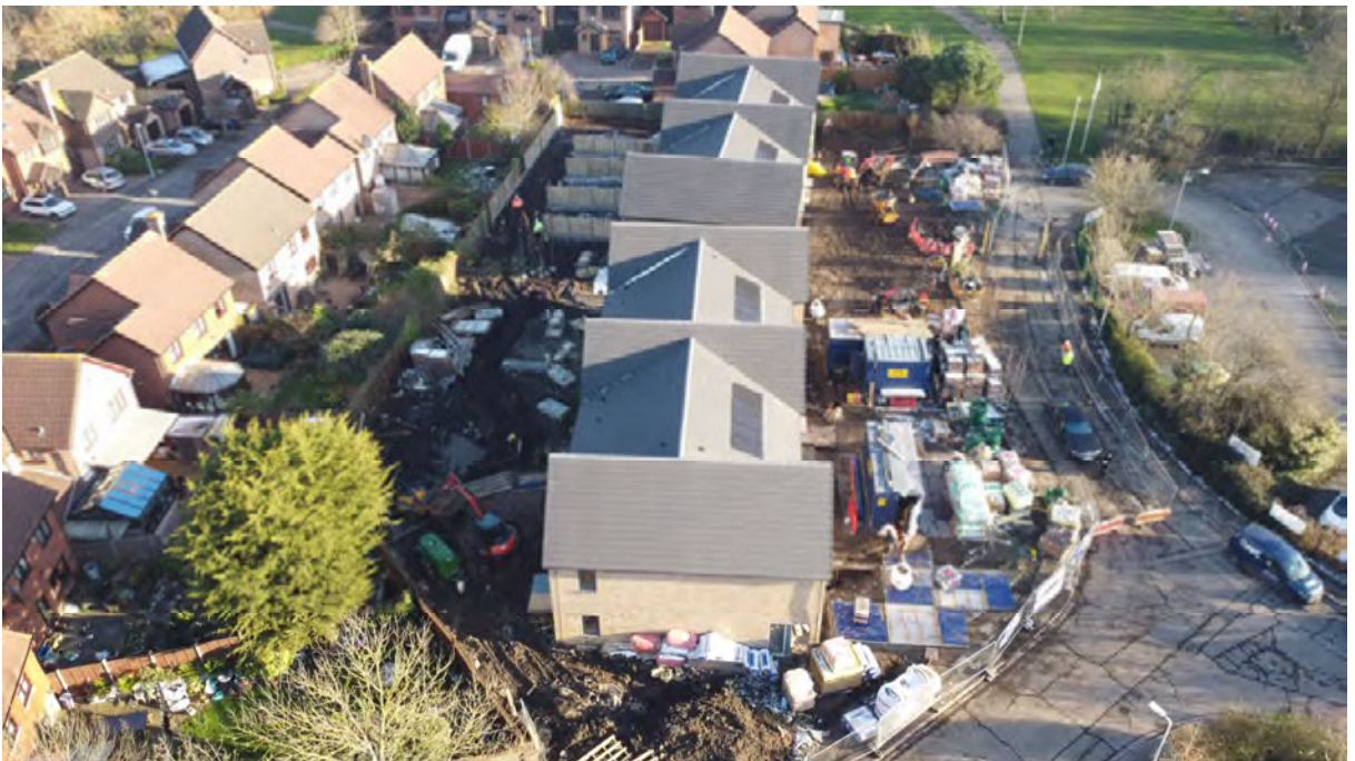
Photograph 2: General site view.
