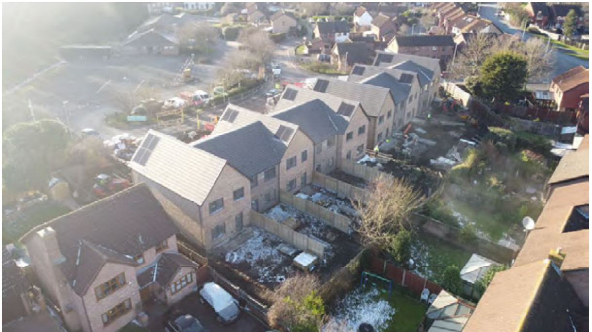
Photograph 6: General site view.
