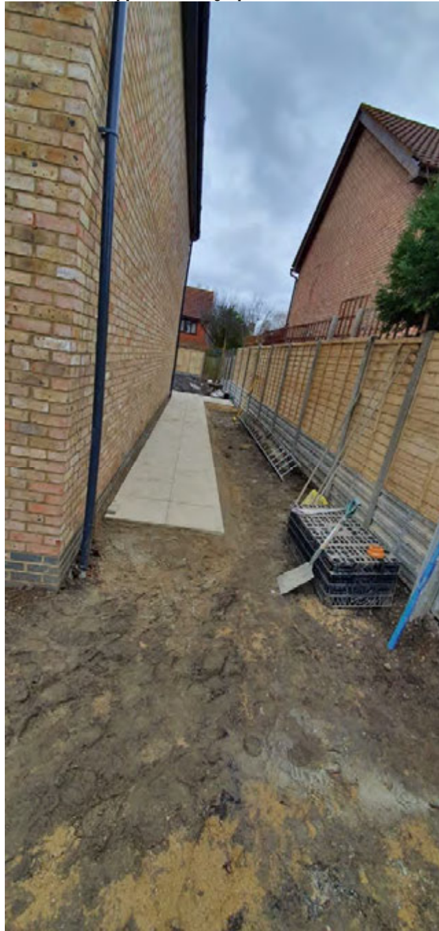
Photograph 30: View of the placement of hardstanding within Plots 6-10.
