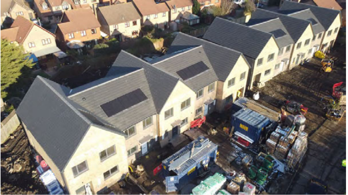
Photograph 1: General site view.
