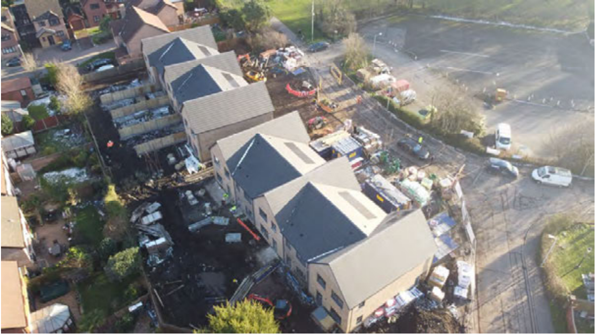
Photograph 3: General site view.
