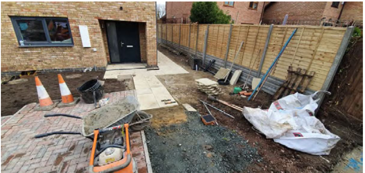
Photograph 34: View of the placement of hardstanding within the front of the properties.
