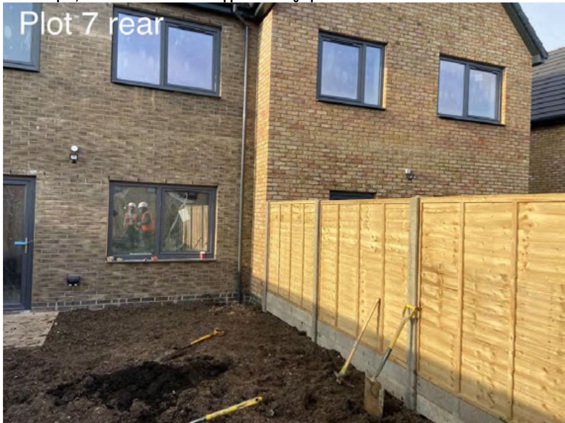
Photograph 16: Verification pit advanced within rear garden of Plot 7.
