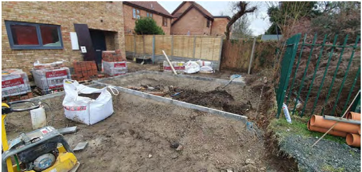
Photograph 25: View of Plots 6-10 prior to the placement of hardstanding.
