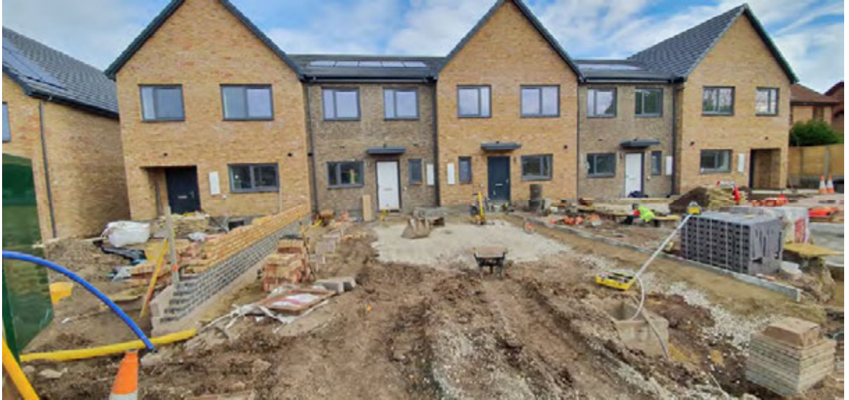
Photograph 33: View of the placement of hardstanding within the front of the properties.
