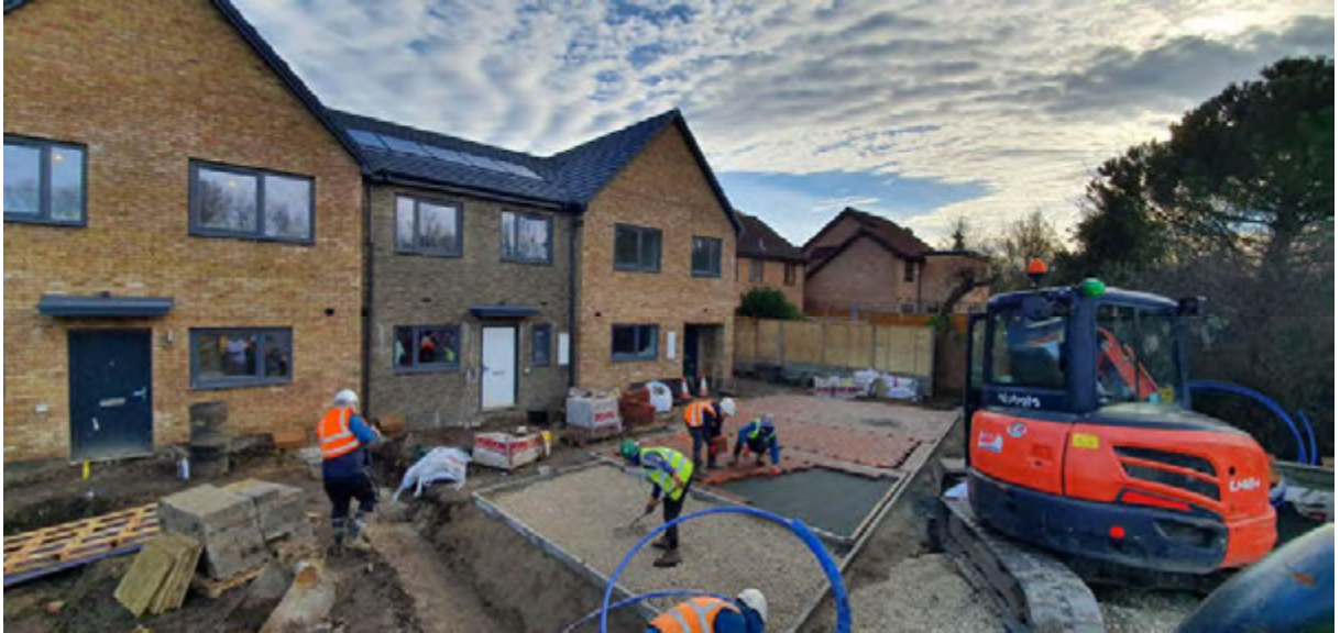
Photograph 31: View of the placement of hardstanding within Plots 6-10.
