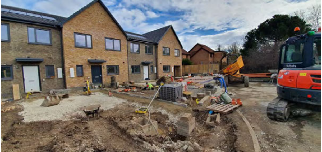
Photograph 37: View of the placement of hardstanding within the front of the properties.
