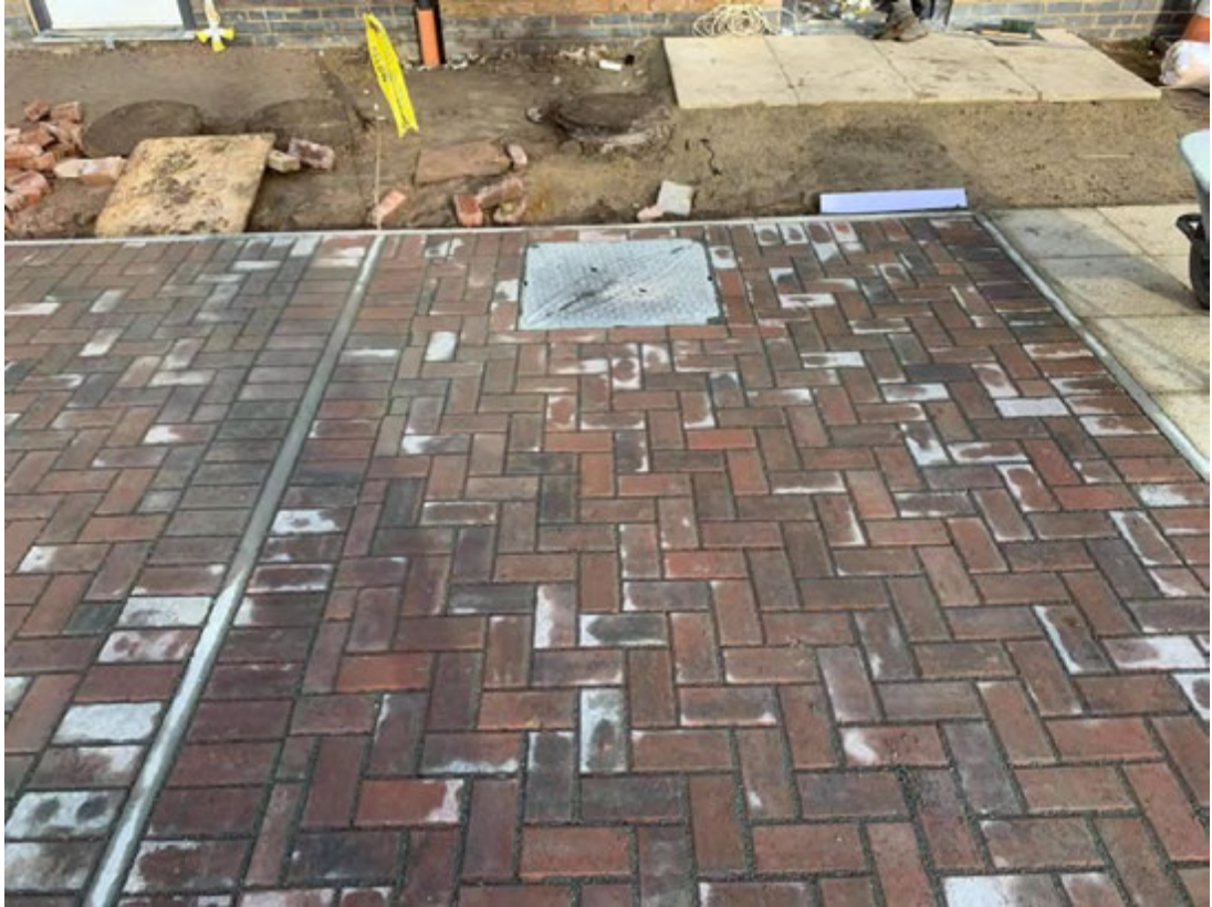
Photograph 24: View of the placement of hardstanding within Plots 1-5.
