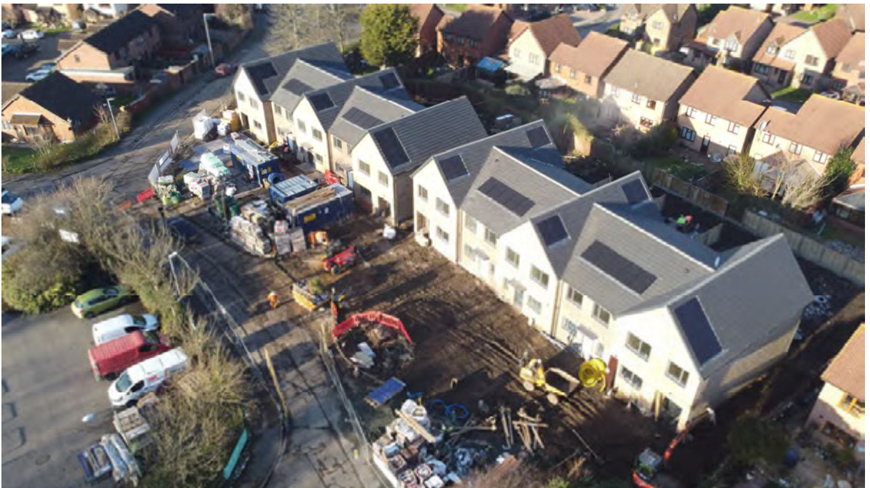
Photograph 8: General site view.
