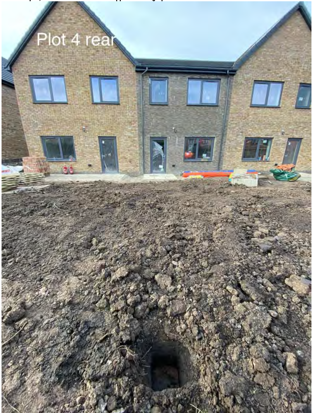
Photograph 14: Verification pit advanced within rear garden of Plot 4.
