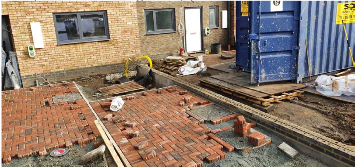
Photograph 18: View of the placement of hardstanding within Plots 1-5.
