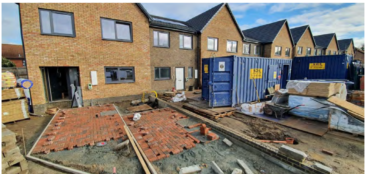
Photograph 20: View of the placement of hardstanding within Plots 1-5.
