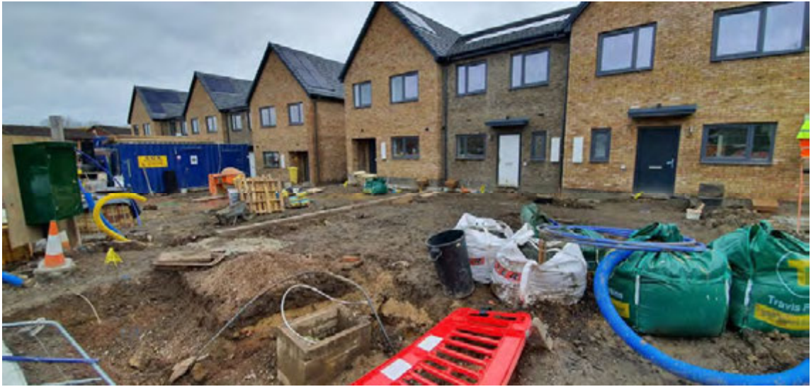
Photograph 28: View of Plots 6-10 prior to the placement of hardstanding.
