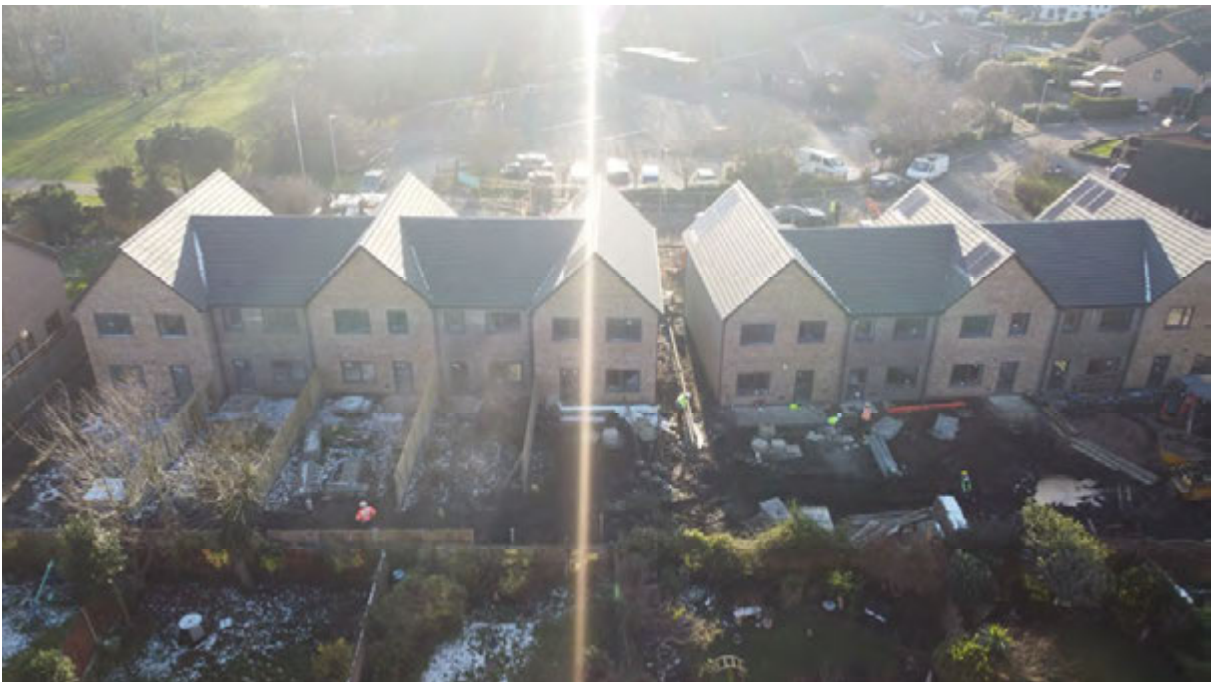
Photograph 4: General site view.
