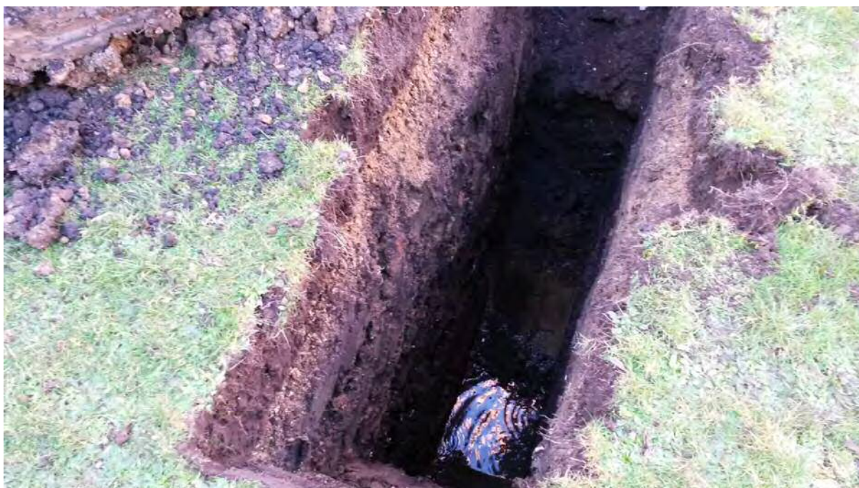
Photograph 5: View of TP03.
