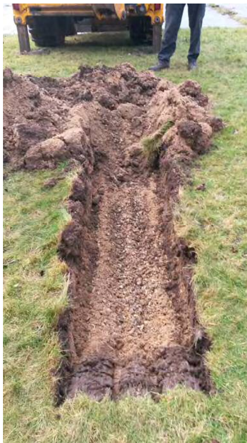
Photograph 1: View of TP01.
