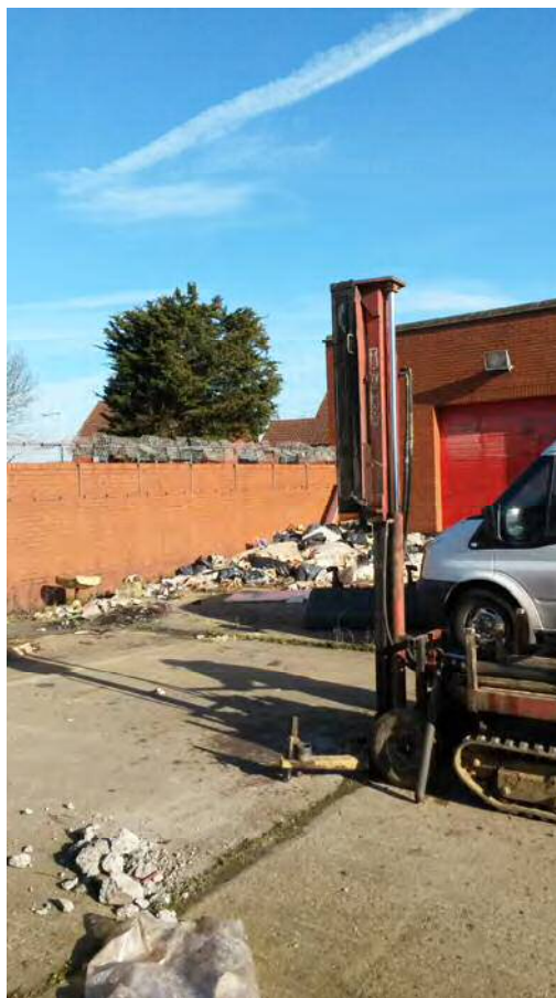
Photograph 7: Location of WS01.
