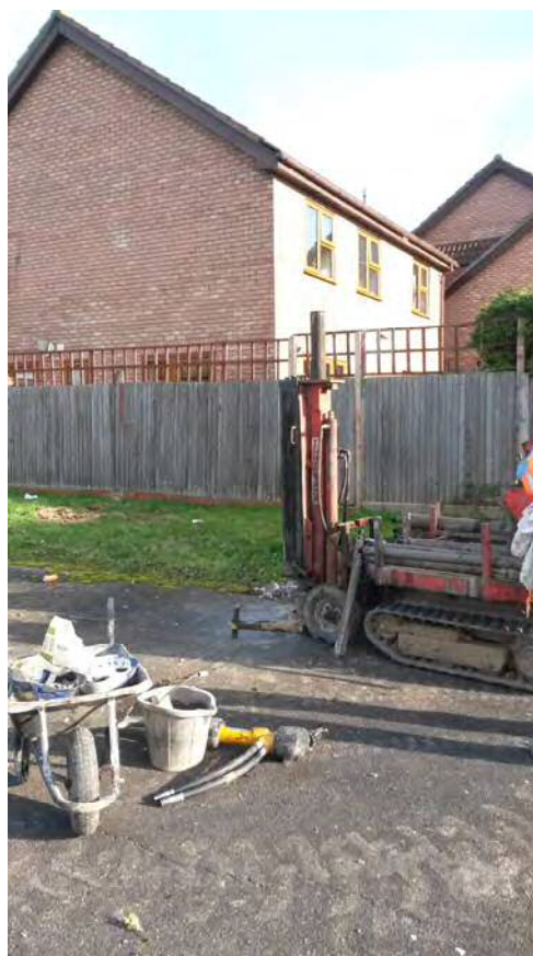
Photograph 12: Location of WS04.
