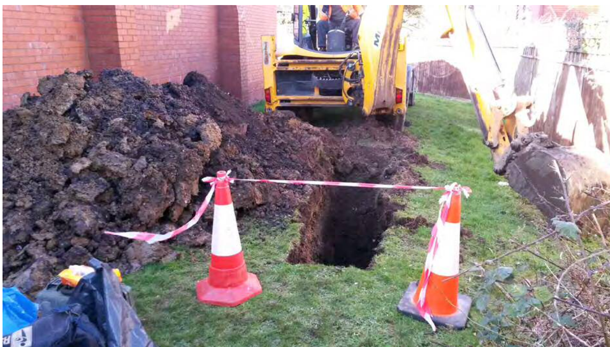
Photograph 4: Location of TP03.
