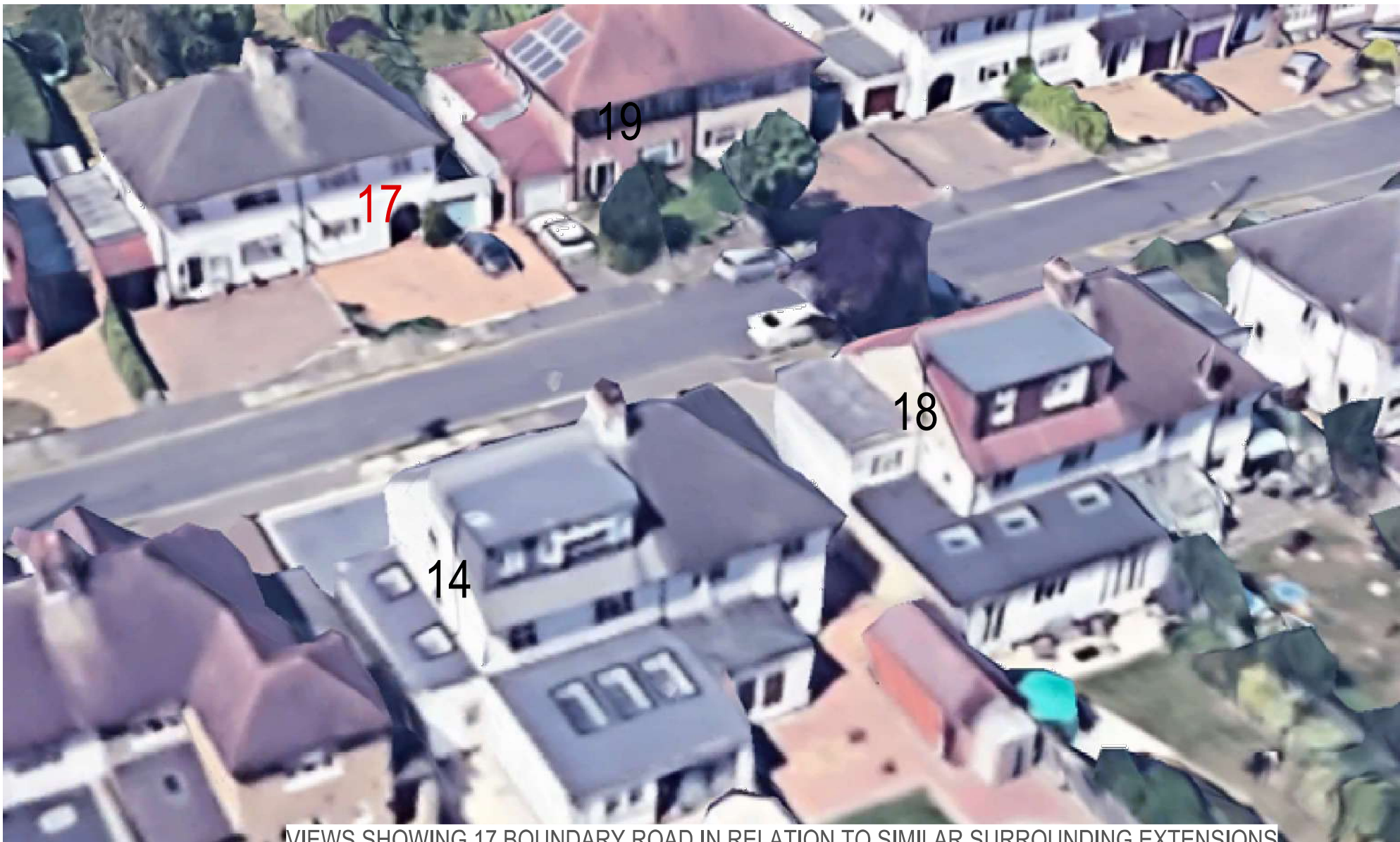
17 VIEWS SHOWING 17 BOUNDARY ROAD IN RELATION TO SIMILAR SURROUNDING EXTENSIONS
