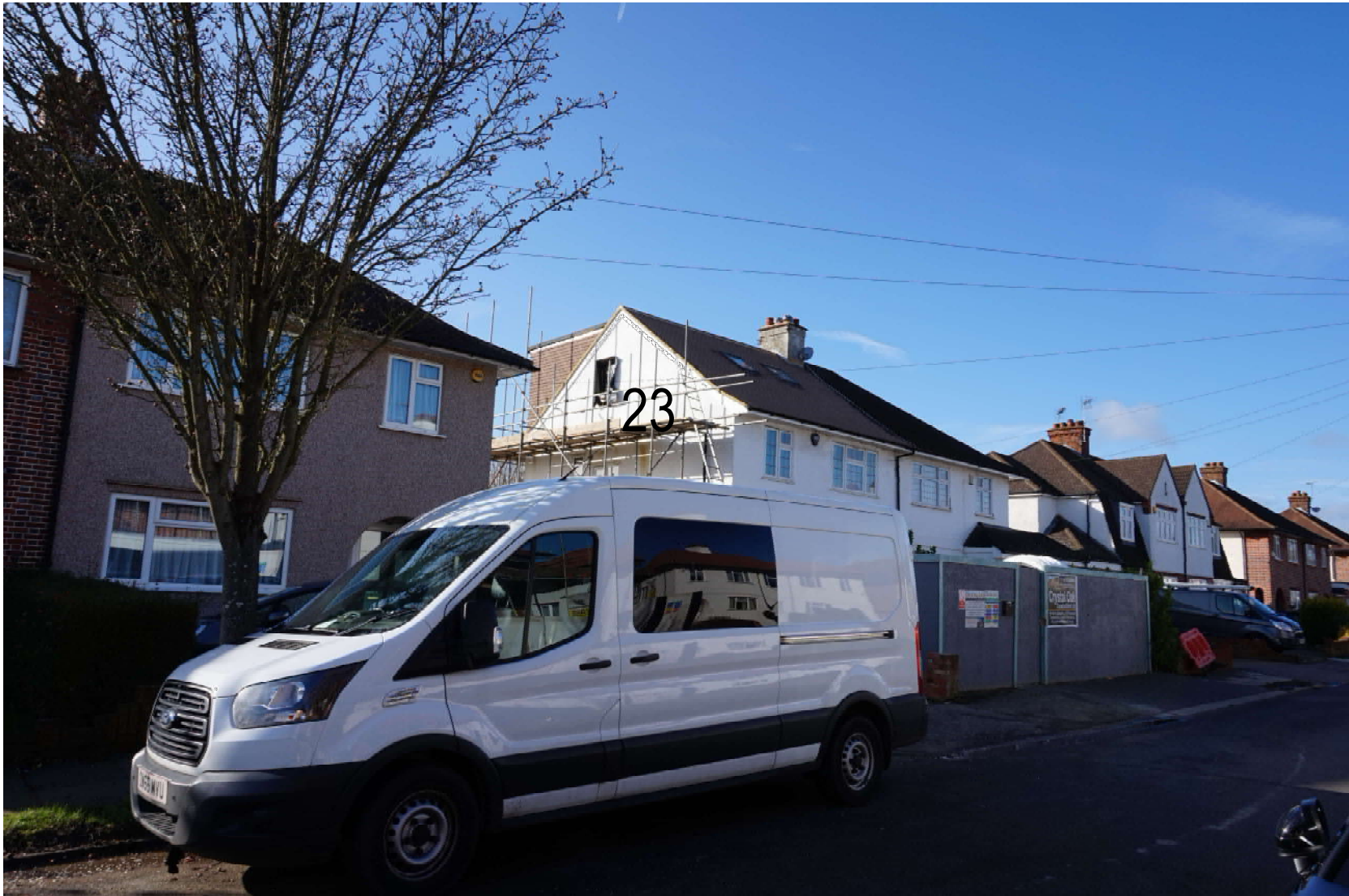
23 VIEW SHOWING 23 BOUNDARY ROAD GABLE END DORMER UNDER CONSTRUCTION
