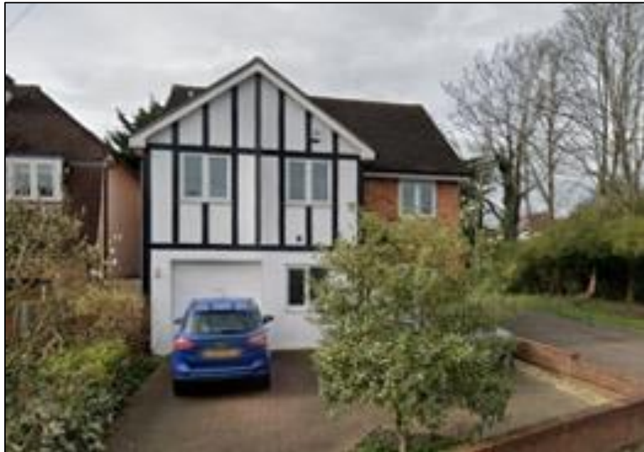
Figure 5: Two storey side extension at The Close/Court Drive Street corner
