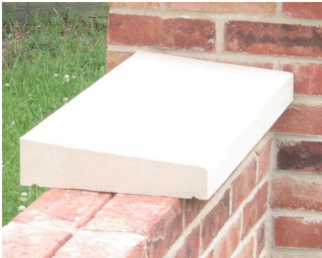
Cast Stone Parapet Coping Plots 1 - 3
