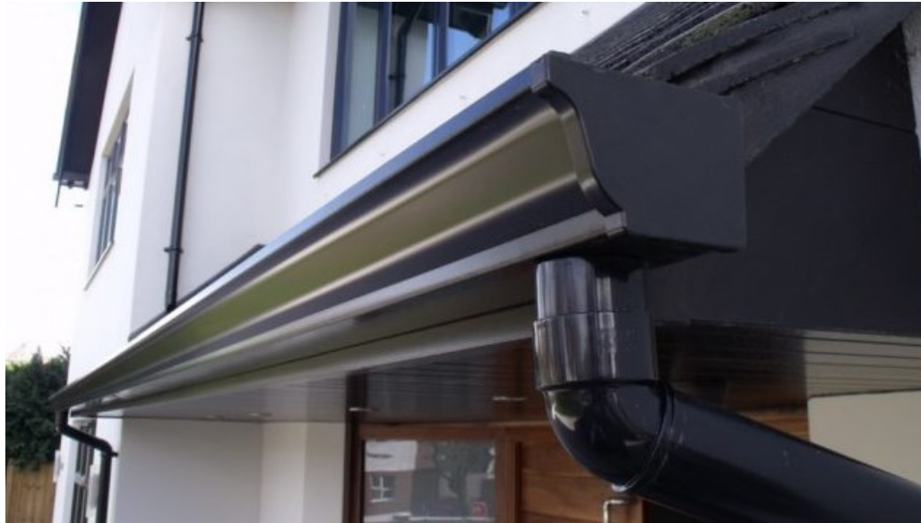
Aluminium gutters and downpipes
