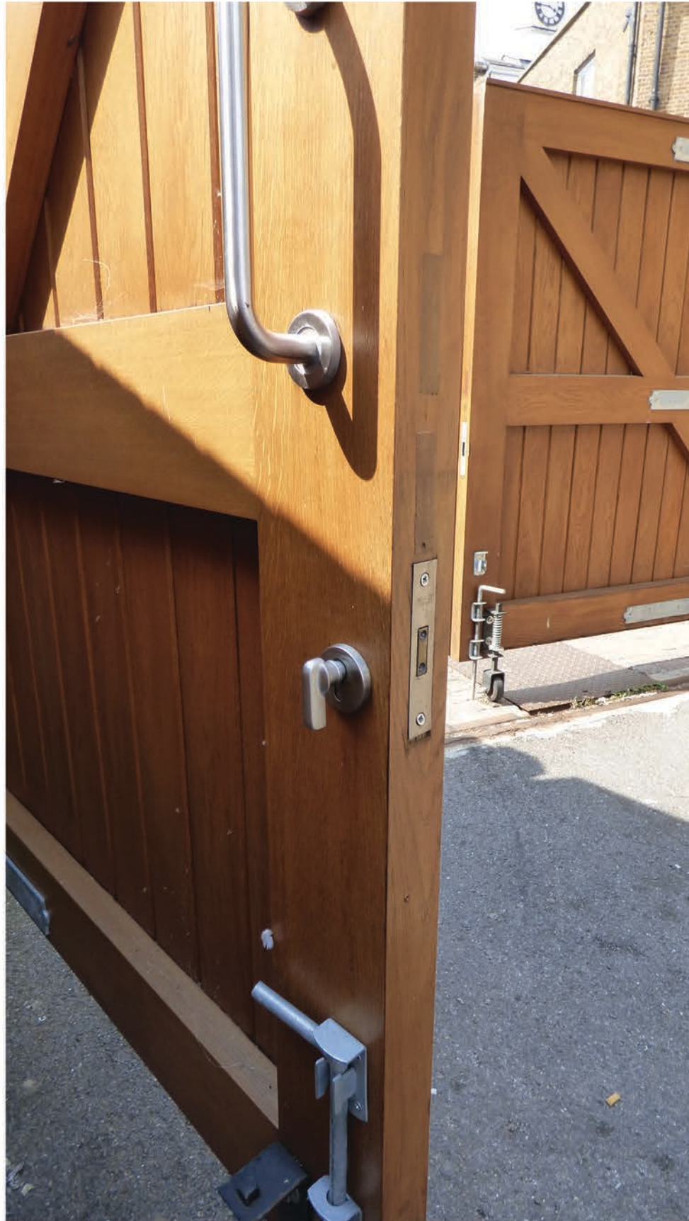
GATE LOCKING MECHANISM
