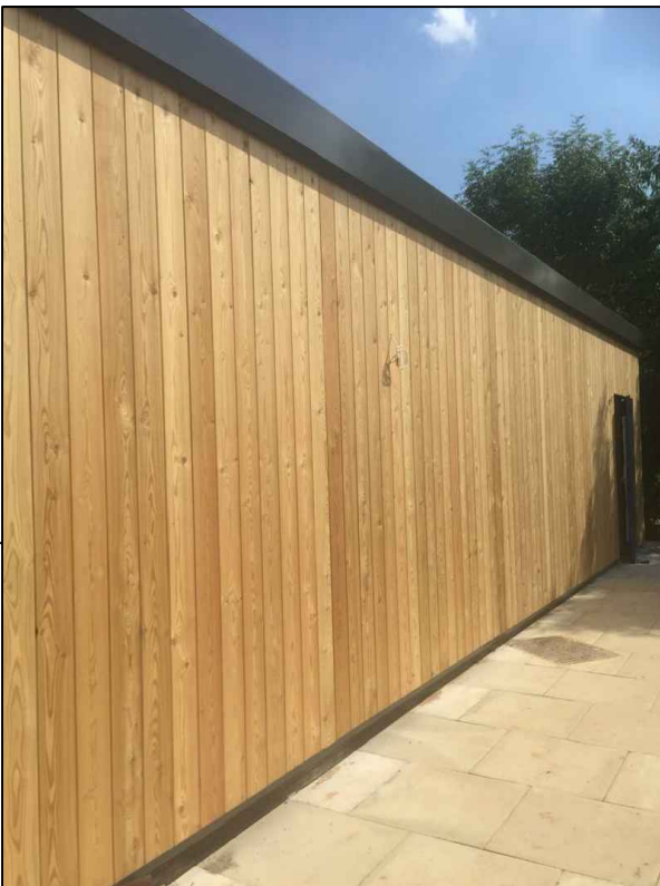
Western Red Cedar No. 2 Clear & Better Tongue & Groove V-Joint vertical timber cladding Board size: 18x94mm, 18x144mm. Grade: No. 2 Clear & Better - 85% Profile: Tongue & Groove connection with a bevelled edge to create a v-shaped shadow line. Surface texture: Smooth.
