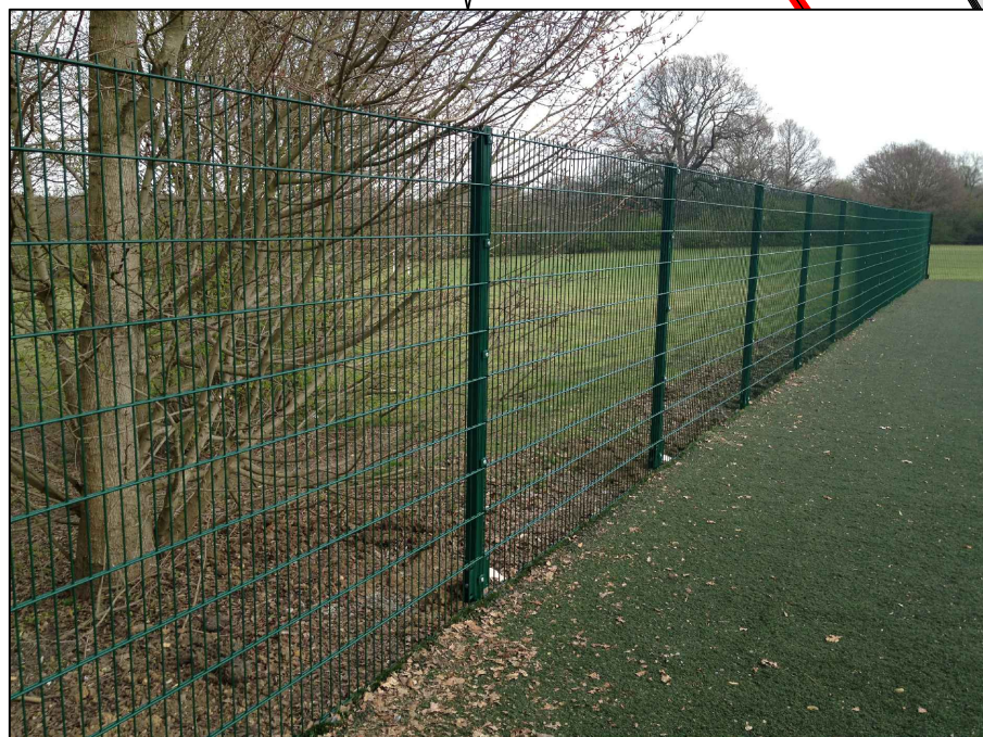
2.4m high green mesh fence Mesh fencing is pre galvanised as well as powder coated RAL 6005 Green
