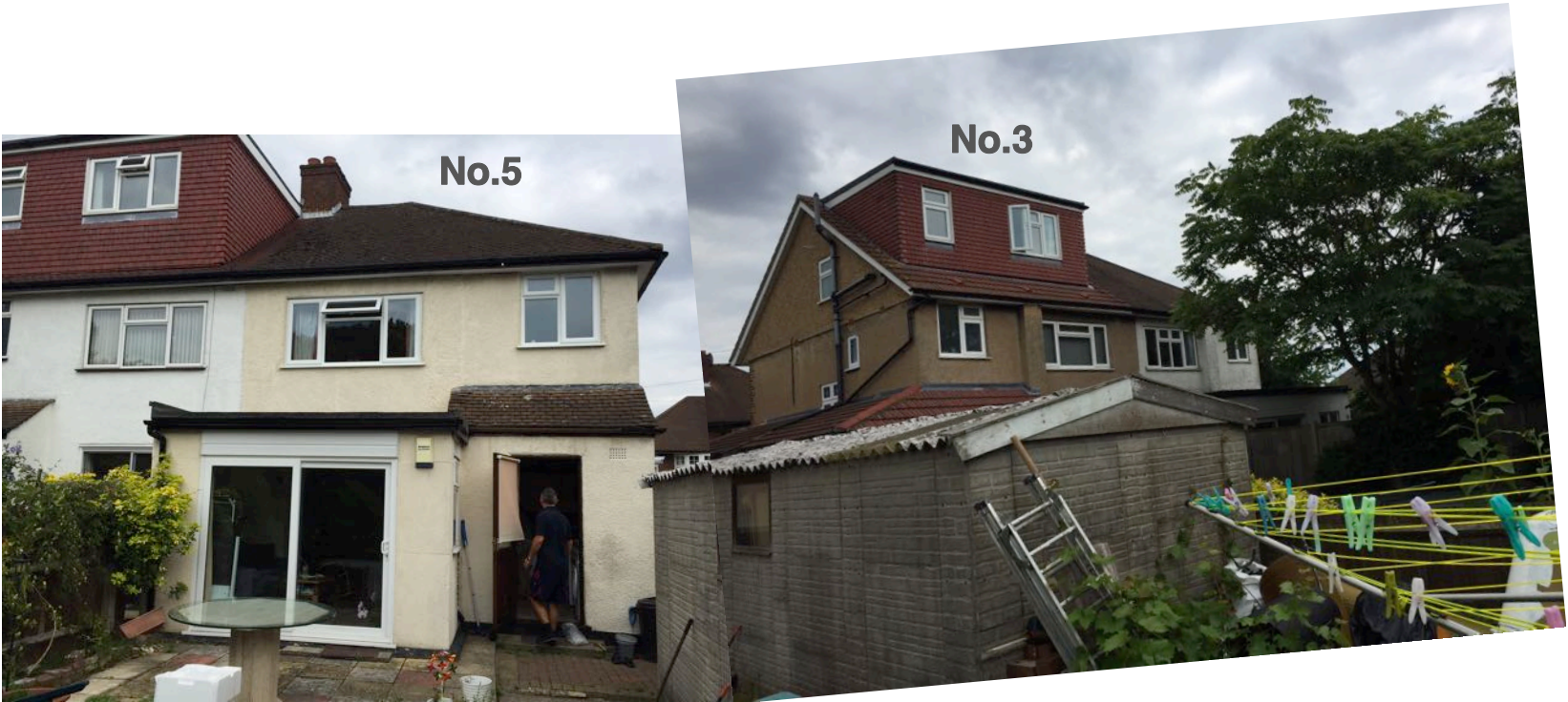
REAR ELEVATION PHOTO
