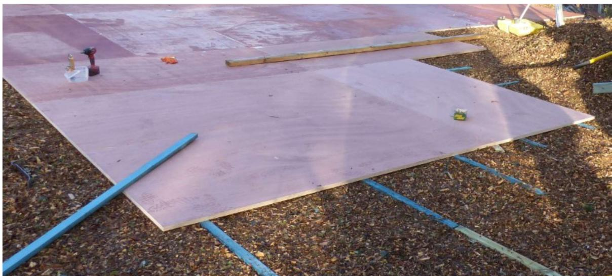
Ply-boards placed onto a layer of woodchips provides a good working surface for pedestrians or scaffolding
