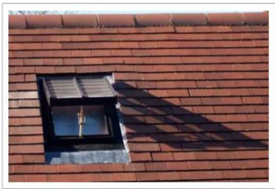
External view to flush installed rooflight
