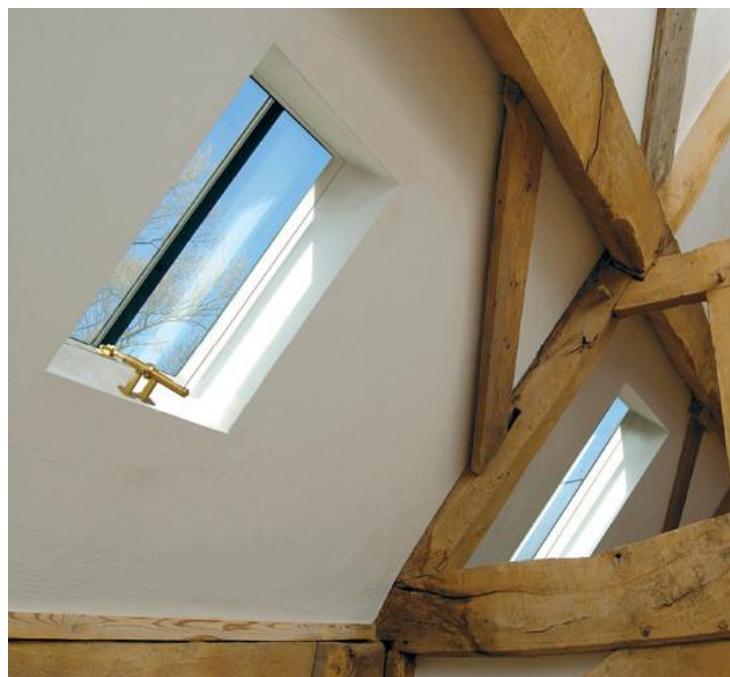
Internal view to flush installed rooflight
