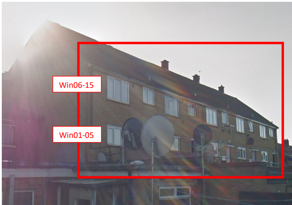
Figure 3 – Neighbouring Windows at No 288-302 High Street (numbering is from left to right)
