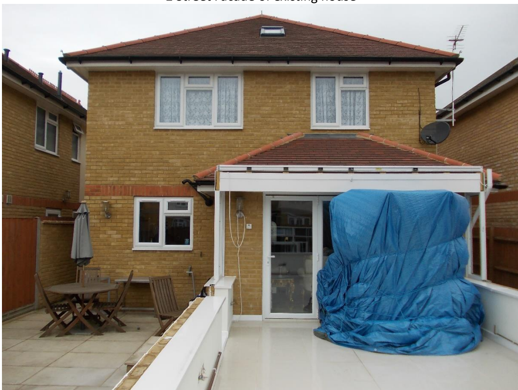
3 Rear of existing house
