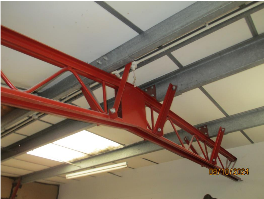
Photograph 10 Internal view of metal truss and purlins.
