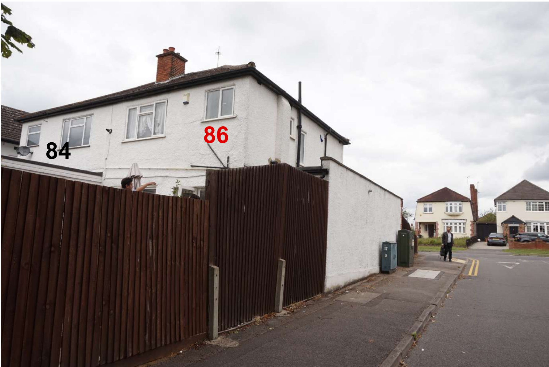
REAR AND SIDE VIEW Showing 86 Bridle Road and 84 Bridle Road (with 3.2M extension) from Rushdene Road
