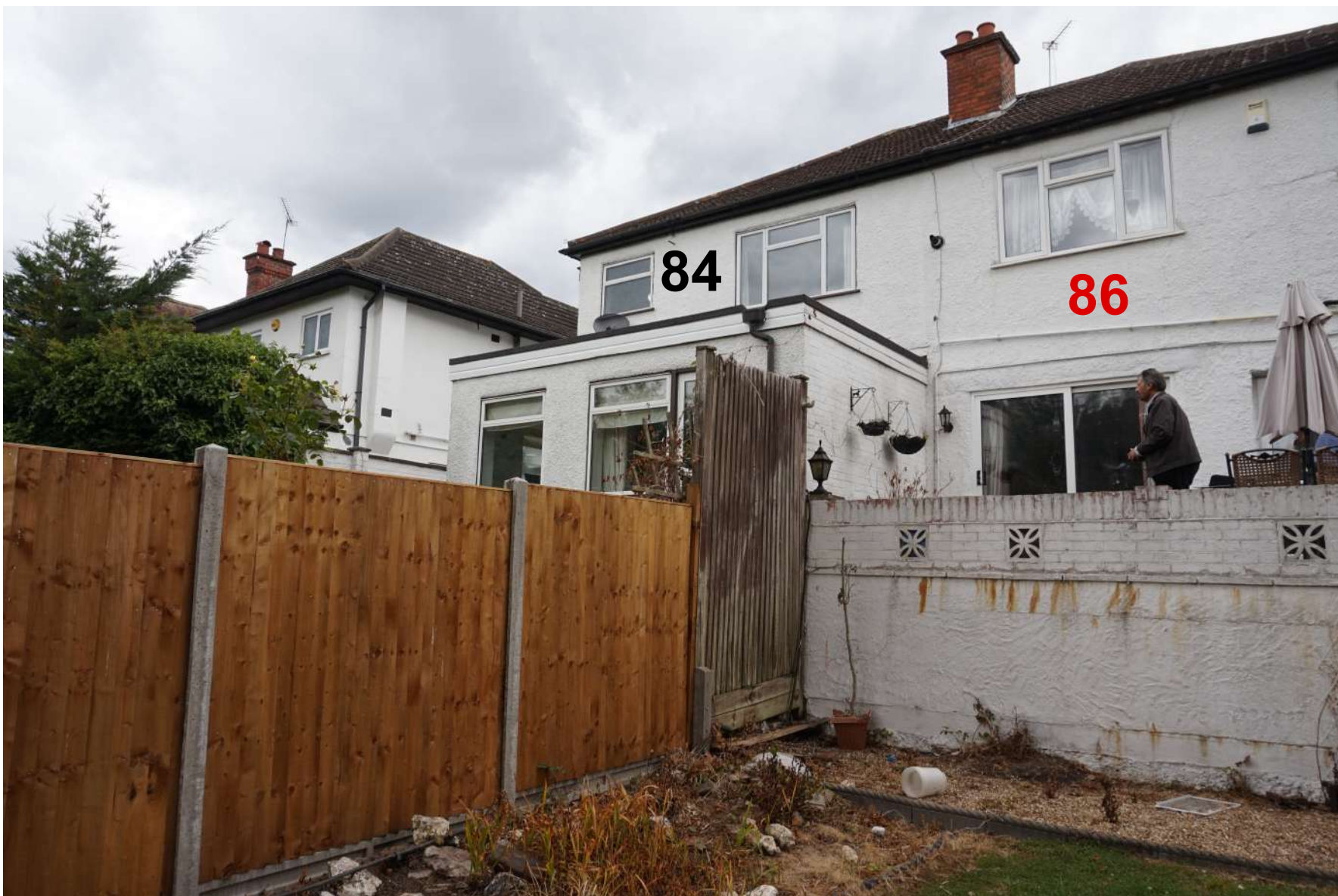
REAR VIEW Showing 86 Bridle Road and 84 Bridle Road (with 3.2M extension) from garden of 86
