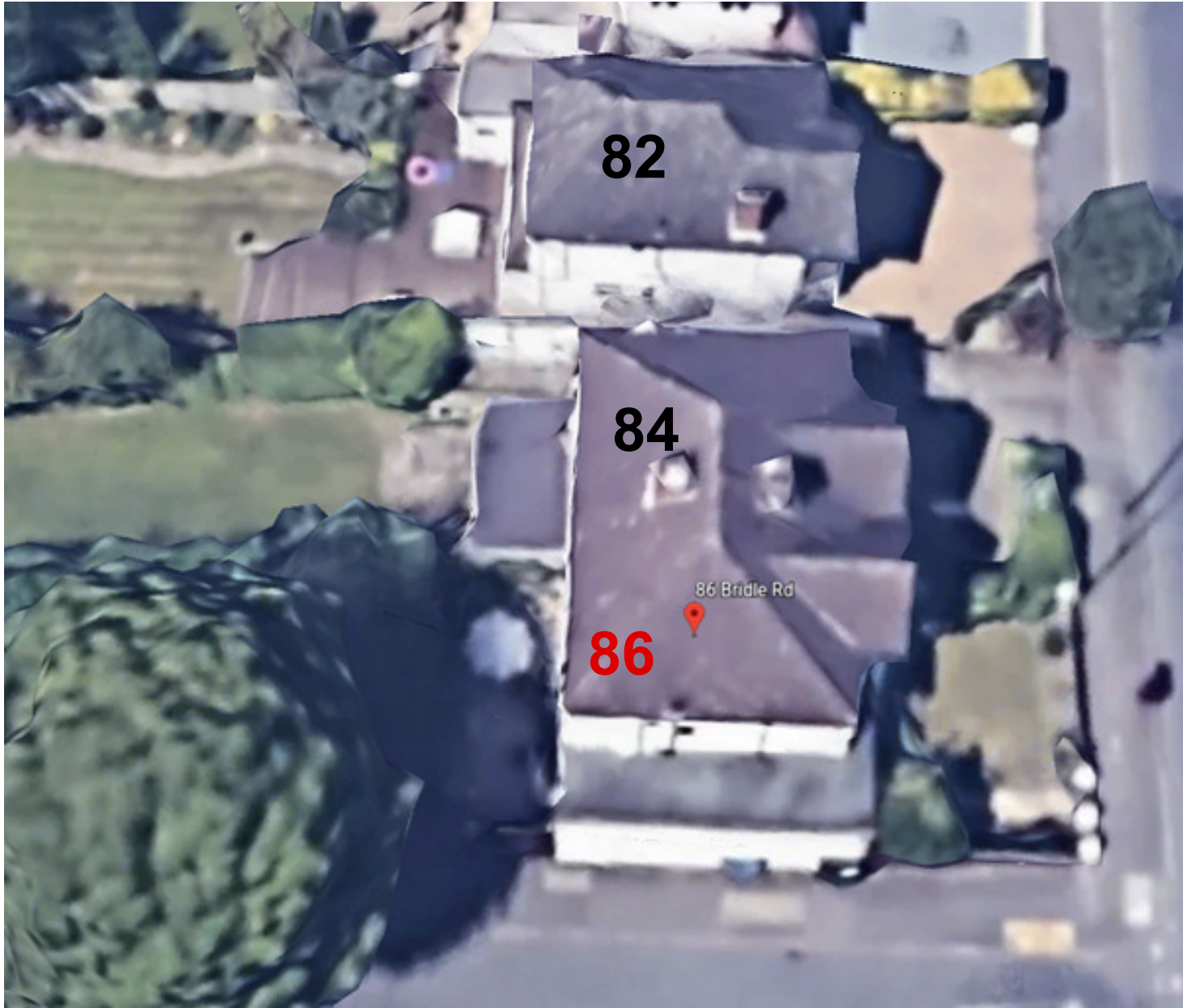
REAR AND SIDE VIEW Showing 86 Bridle Road and 84 Bridle Road (with 3.2M extension) 82 Bridle Road (with elevated decking area extending out into garden)
