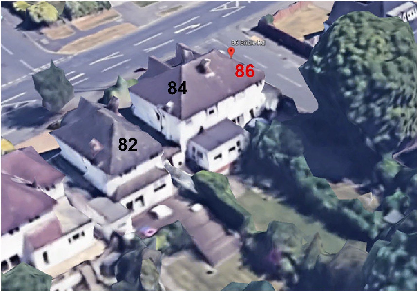
REAR AND SIDE VIEW Showing 86 Bridle Road and 84 Bridle Road (with 3.2M extension) 82 Bridle Road (with elevated decking area extending out into garden)
