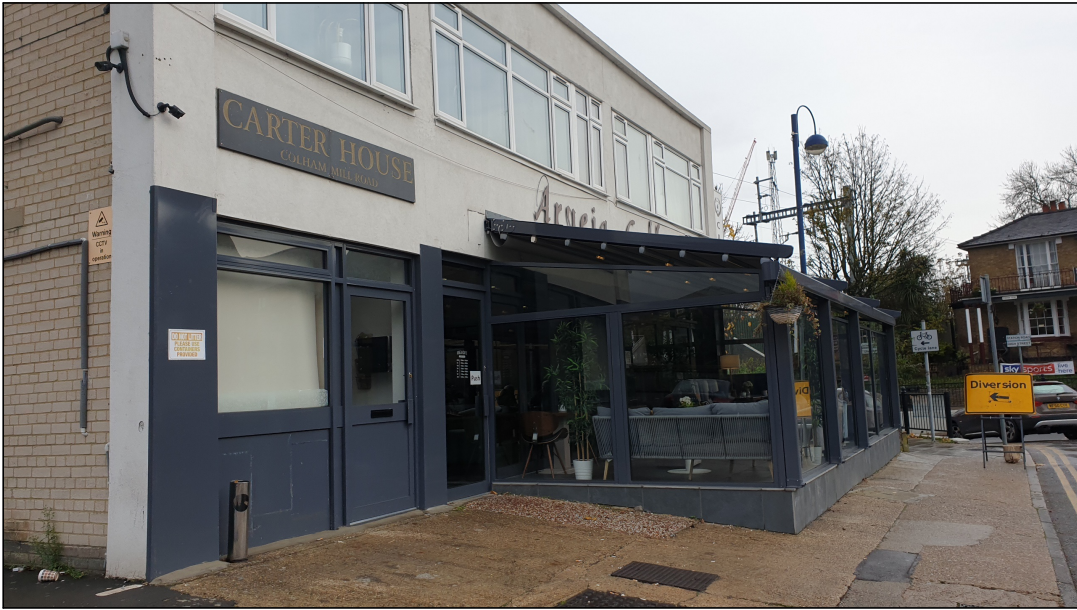
EXISTING SIDE VIEW
