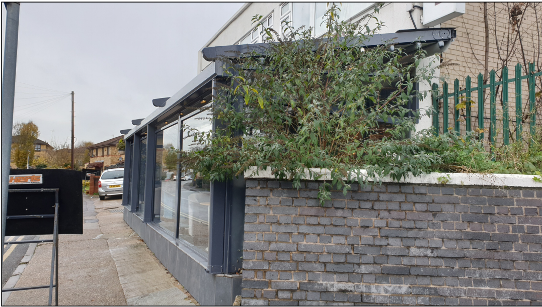
EXISTING SIDE VIEW
