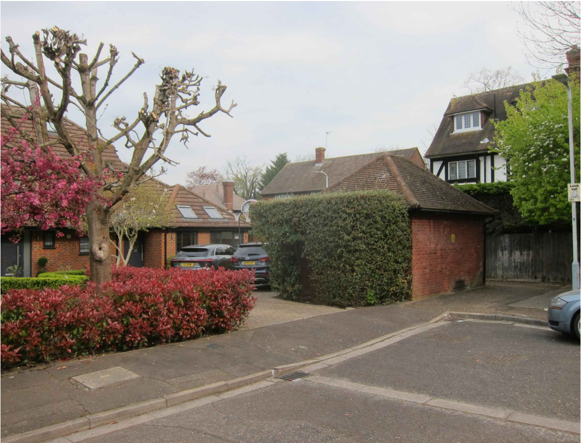
Street View looking right (including UKPN substation)
