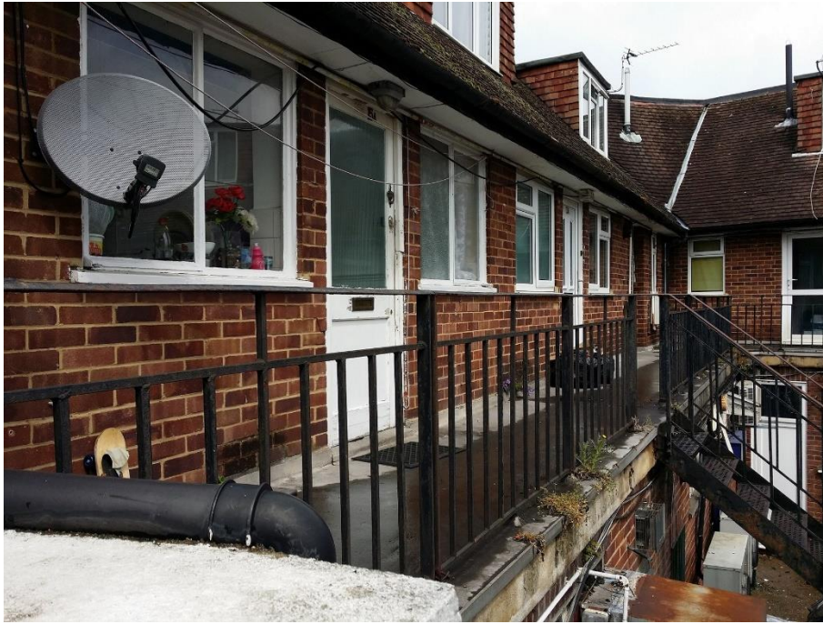
A view of the access walkway serving the adjacent flats
