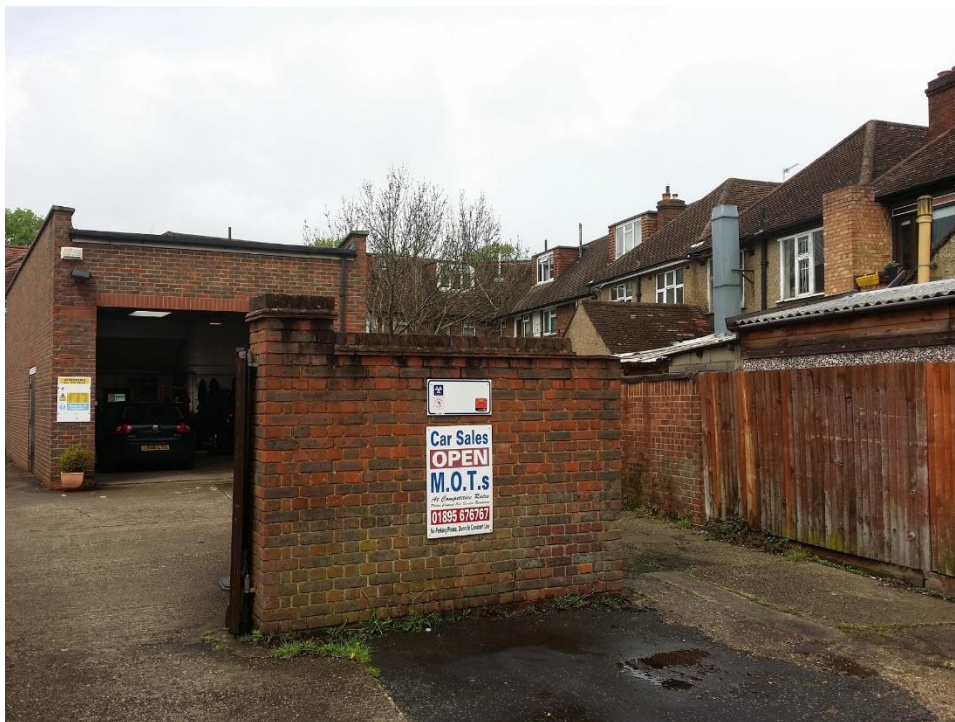
A view from Edinburgh Drive showing the dormers in the roof of adjacent properties
