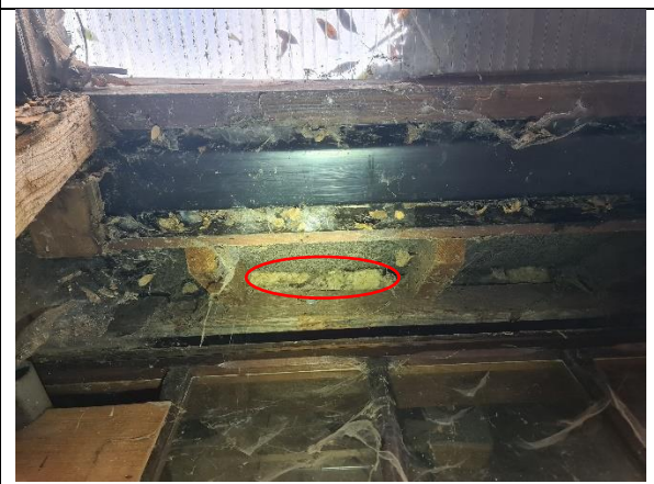
Image 6: Section 2 pitch with expanding foam filling.
