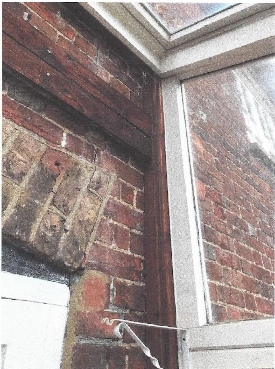
VIEW OF FRONT PRINCIPAL ENTRANCE DOOR OPENING WITH DAMAGED BRICK REVEALS AND BRICK ARCH.
