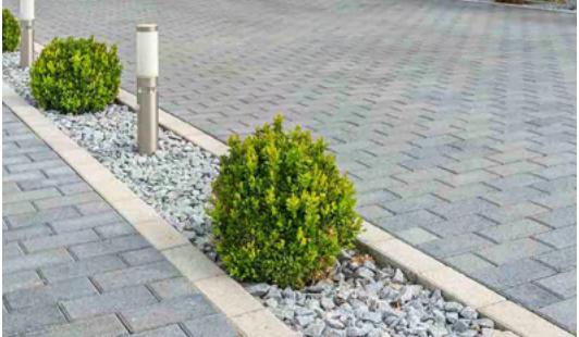
Concrete block paving to private driveways and parking
