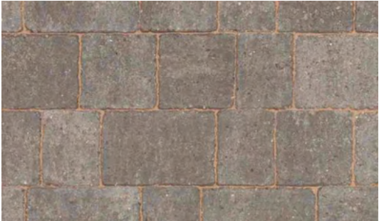
Concrete paving to courtyard garden
