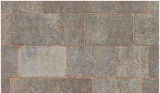
Concrete block paving to main pedestrian pathways
