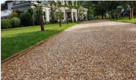
Reinforced gravel secondary driveway and car parking bays
