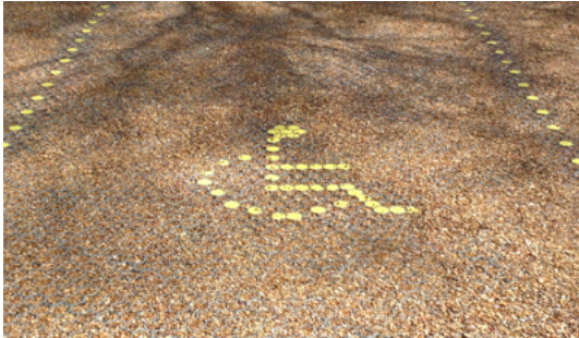
Reinforced gravel to DDA parking spaces with yellow inserts for demarcation
