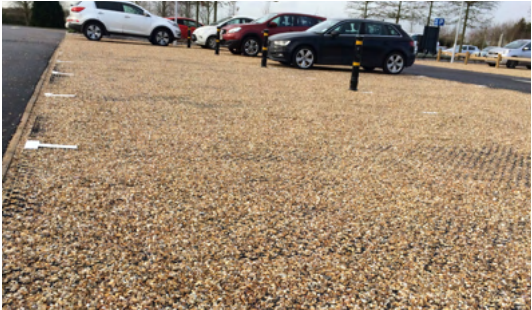
Reinforced gravel to car parking spaces
