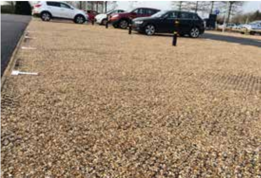
REINFORCED GRAVEL TO CAR PARKING SPACES
