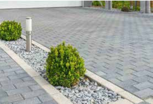
CONCRETE BLOCK PAVING TO PRIVATE DRIVE WAY AND PARKING
