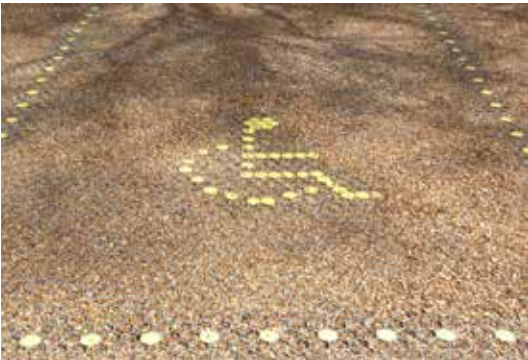
REINFORCED GRAVEL TO DDA PARKING WITH YELLOW INSERTS FOR DEMARCATION
