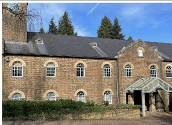
B1 Stable building
