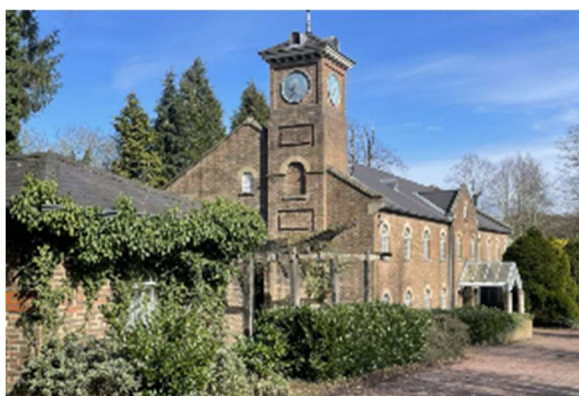
B1 Stable building
