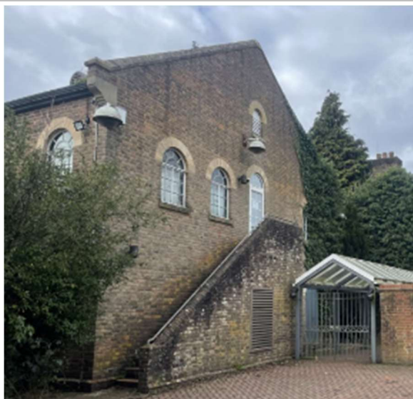
B1 Stable building
