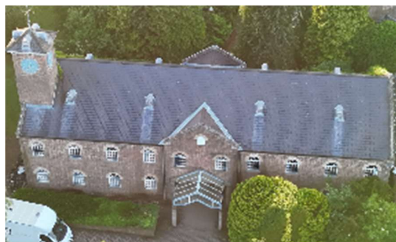
B1 Stable building
