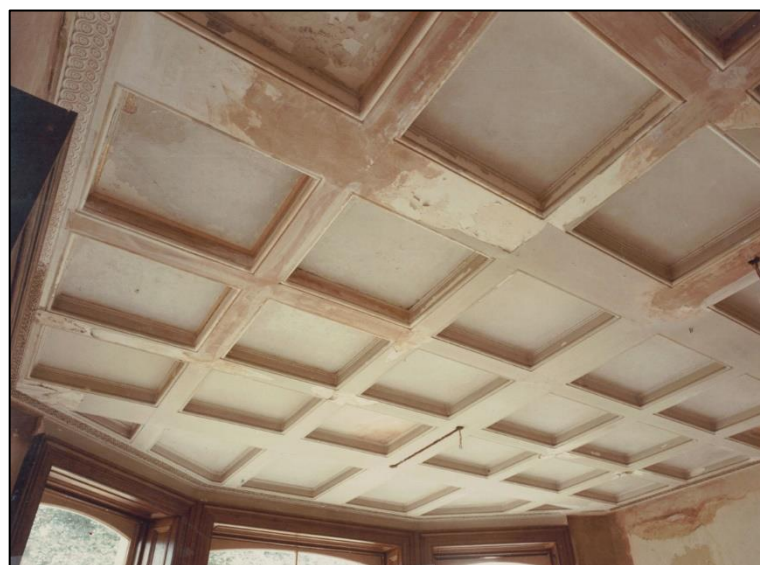
Figure 27: The almost complete coffered ceiling
