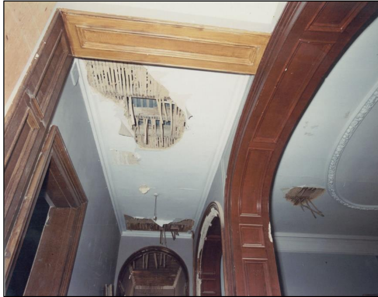
Figure 23: The lath and plaster ceiling, cornice and arch details in G1/G2 in 1983
