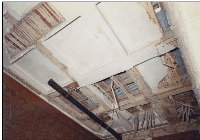
Figure 26: The coffered ceiling in G6 undergoing restoration in 1983
