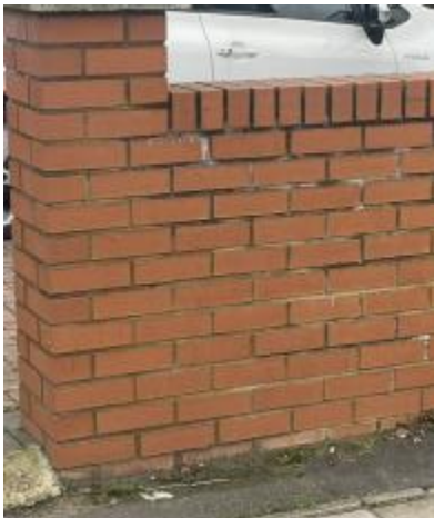
Low Brick Wall
