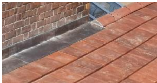
8 Code 5 Lead Flashing
