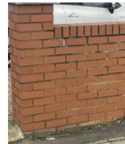
Low Brick Wall
