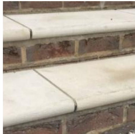
Pave Stone Step Bull Nose
