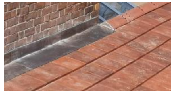
8 Code 5 Lead Flashing
