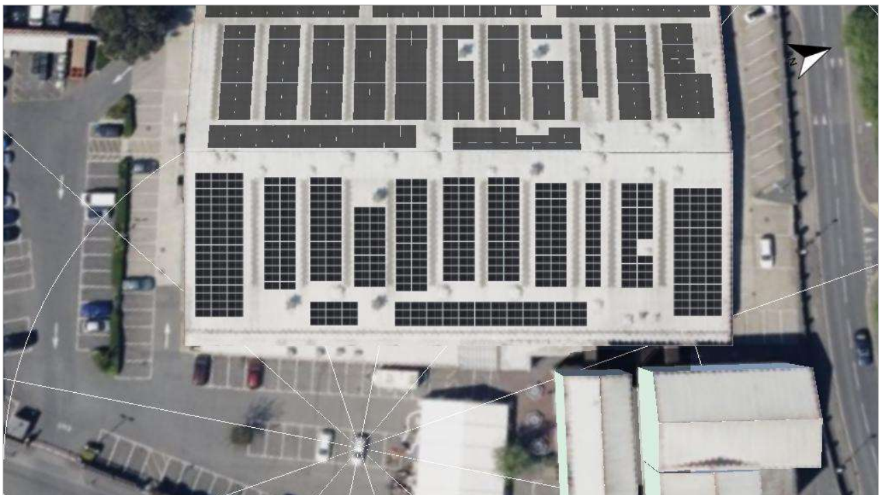
Figure: 1. Module Area - Building 13-Roof Area East
