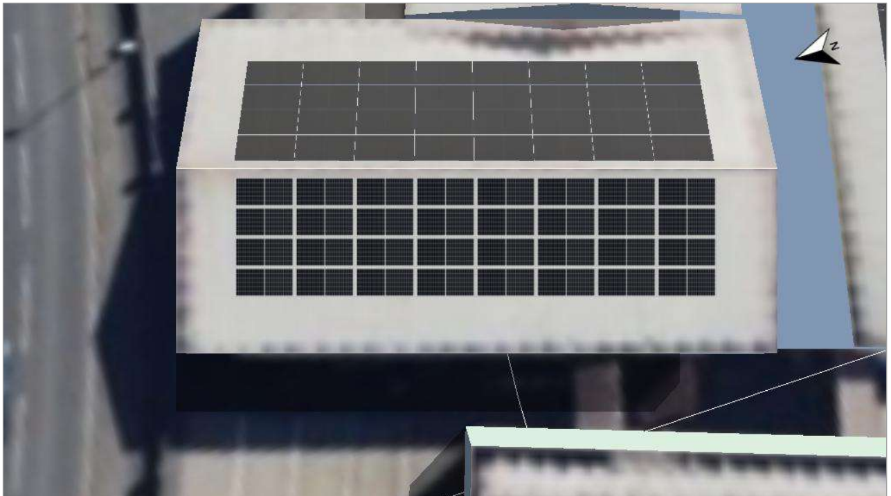
Figure: 6. Module Area - Building 12-Roof Area West
