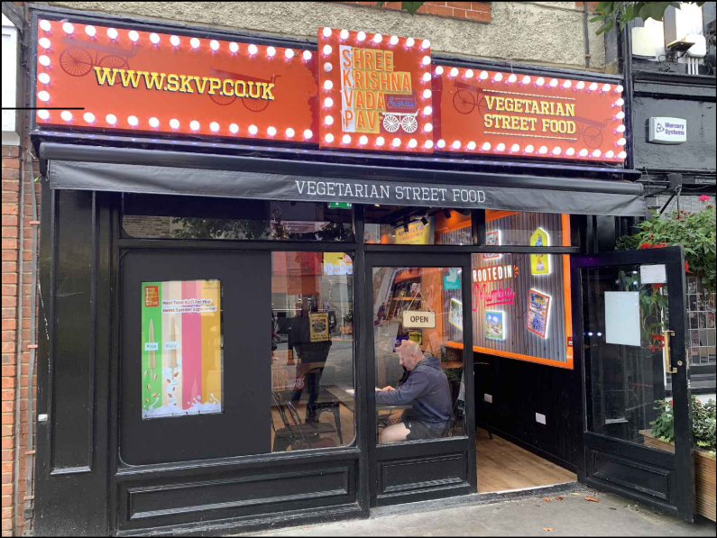
Photo of shop front with sign and awning over
