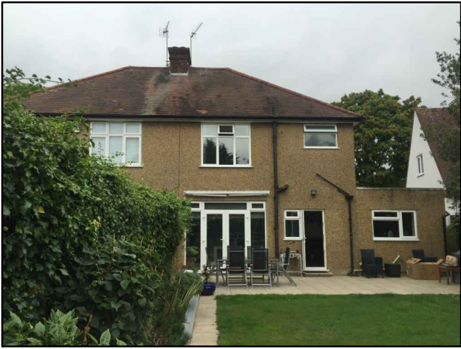
Photo Showing Existing Rear Elevation
