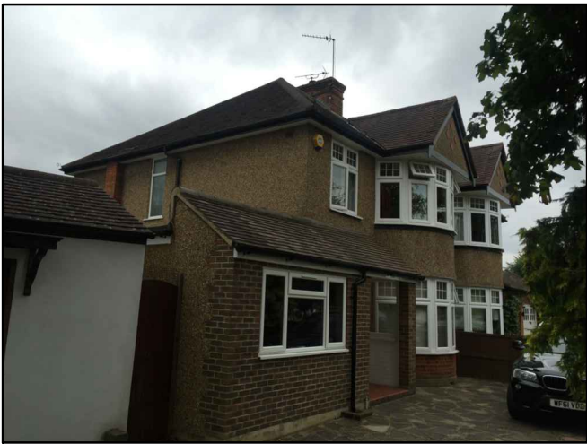
Photo Showing Existing Front Elevation
