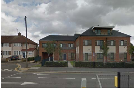
1. Housing development in the corner of Station Approach and West End Road.
