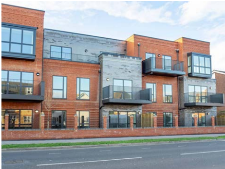
Acol Crescent Development - from site
