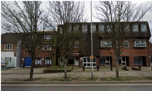
1. Morritt House, on the corner between Station Approach and Deane Avenue.
