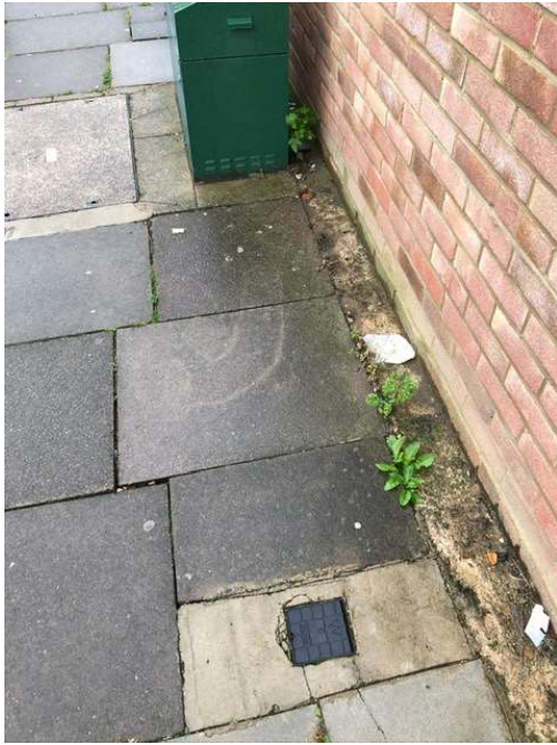
Figure 3 – Evidence of services on Northolt Avenue side of property
