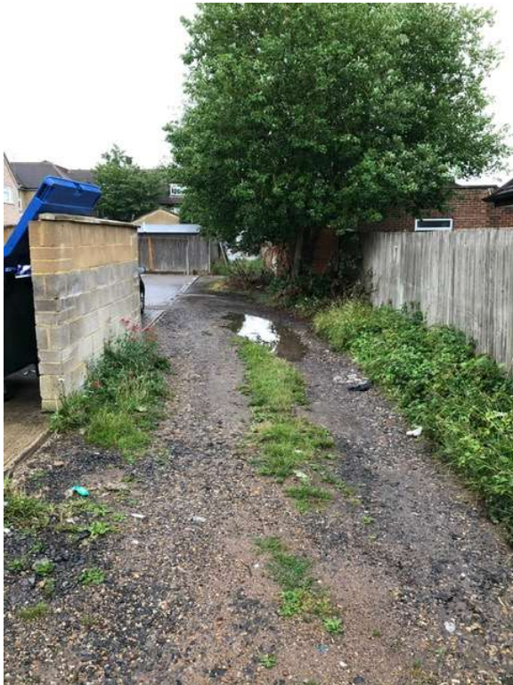
Figure 6 – Rear service track
