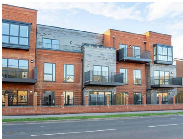
Acol Crescent Development - from site
