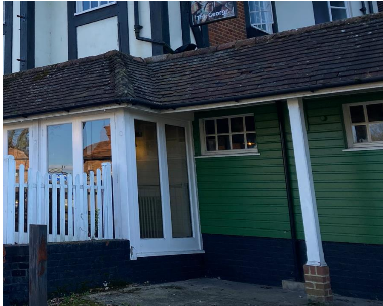
Existing timber weather board cladding
