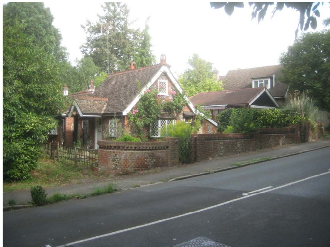
Ducks Hill Road - Rustic Cottage (listed building)
