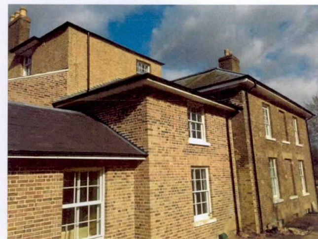
Plate 11: Side/rear elevation of Manor Court
