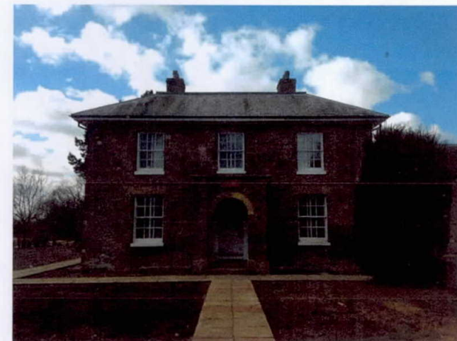
Plate 10: Front elevation of Manor Court
