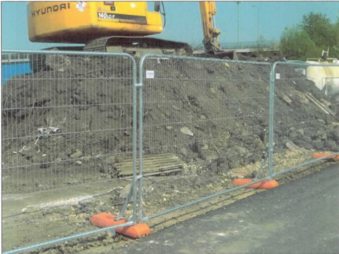
Photograph D - Tree Protective Fencing
