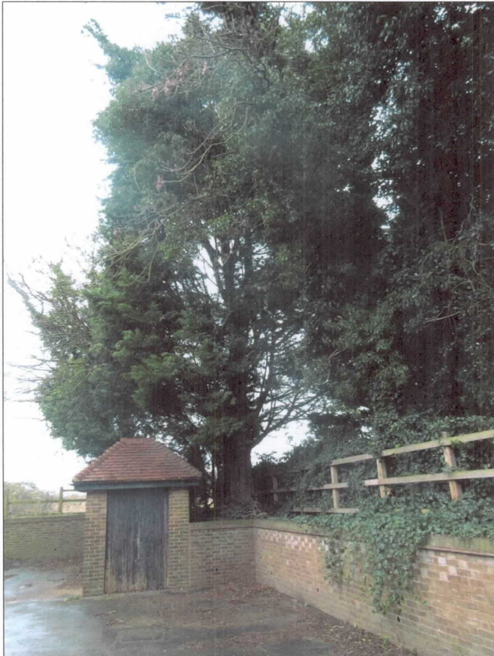
Photograph E – Looking north towards G3, G4 and Ash (T2) all situated in an area retained by a brick retaining wall.
