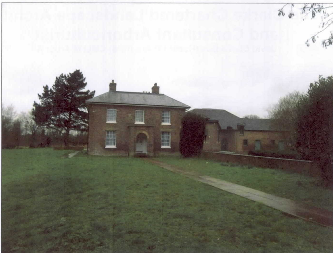
Photograph A – looking west from within the site towards Manor Court one the buildings within the site.
