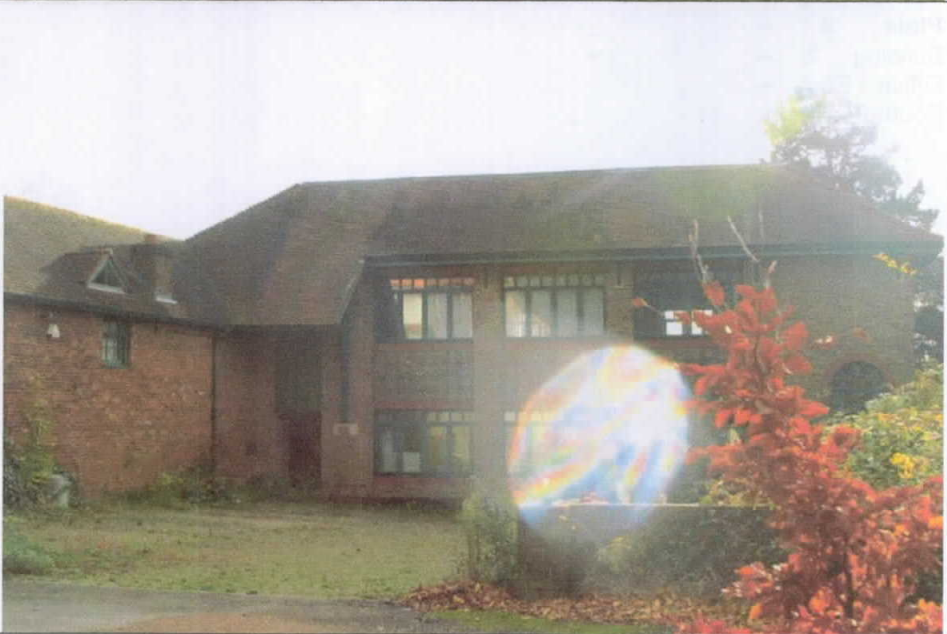
Plate 6 – Extension of rear elevation of Building 2 – Former Stable Block
