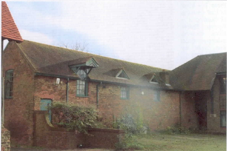
Plate 5 – Rear elevation of Building 2 showing small dormers
