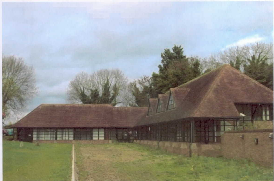
Plate 10 – Building 3 Office Barn west and south elevations
