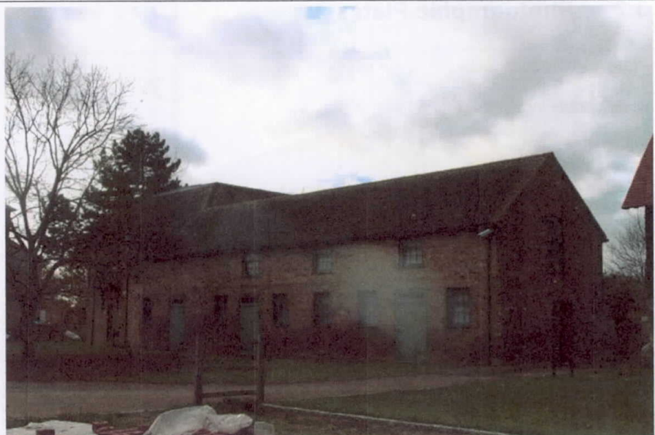
Plate 3 – Building 2 – Former Stable Block west facing elevation
