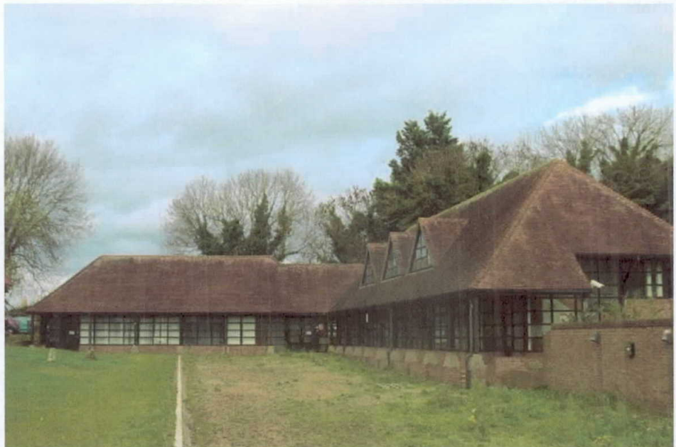
Plate 10 – Building 3 Office Barn west and south elevations
