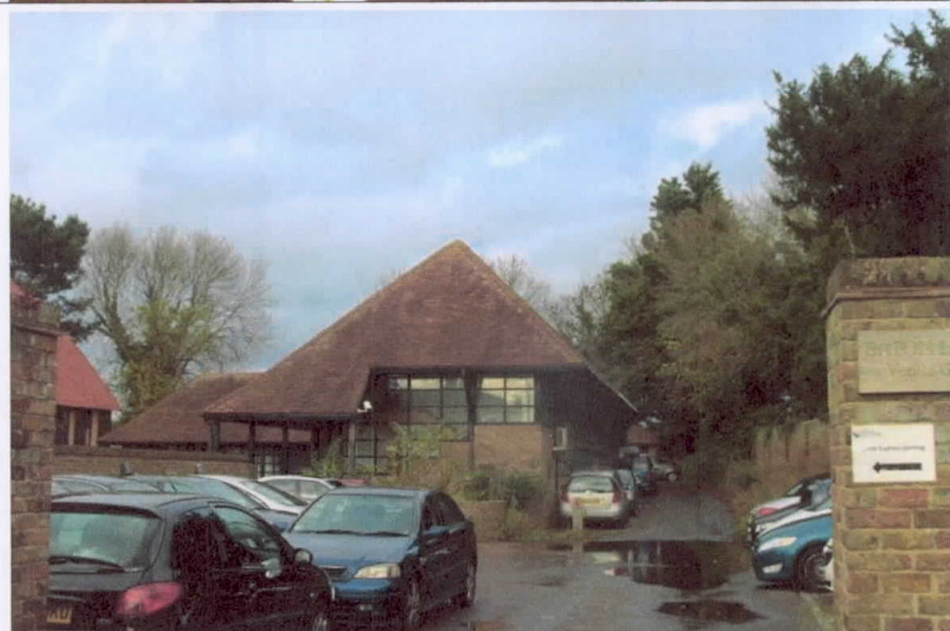
Plate 8 – Building 3 – Office Barn – South Elevation
