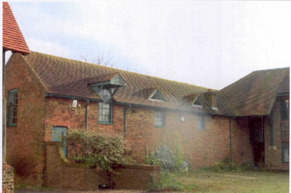
Plate 5 – Rear elevation of Building 2 showing small dormers
