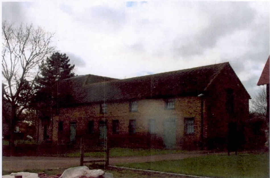
Plate 3 – Building 2 – Former Stable Block west facing elevation
