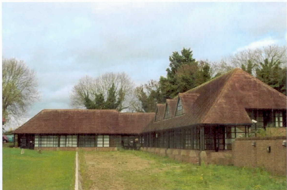
Plate 10 – Building 3 Office Barn west and south elevations
