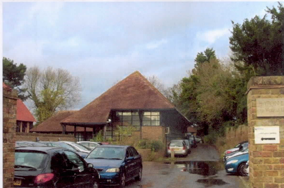
Plate 8 – Building 3 – Office Barn – South Elevation
