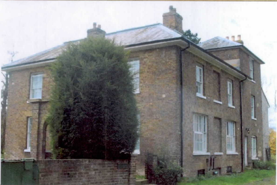
Plate 2 – Building 1 – Manor Lodge – Building with no potential bat access
