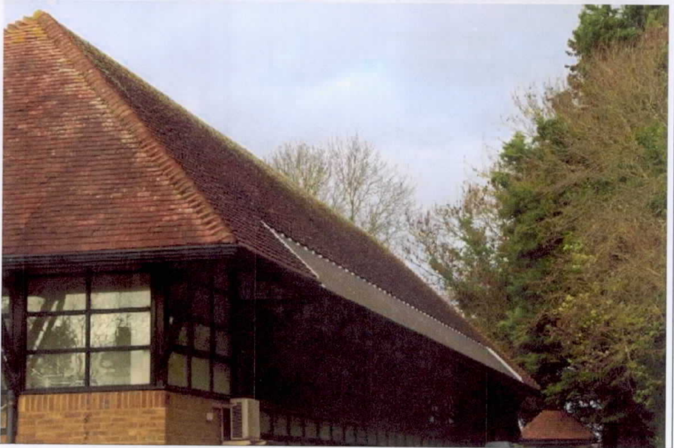
Plate 9 – Office Barn View of East elevation showing corrugated panels along bottom of roof slope
