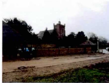
Fig 5: View of St. Mary's Church from within the site
