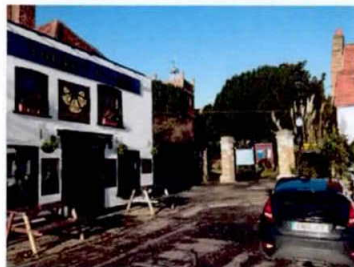
Fig 7: View of Five Bells Public House
