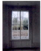
REMOVAL OF INSENSITIVE SECONDARY GLAZING
