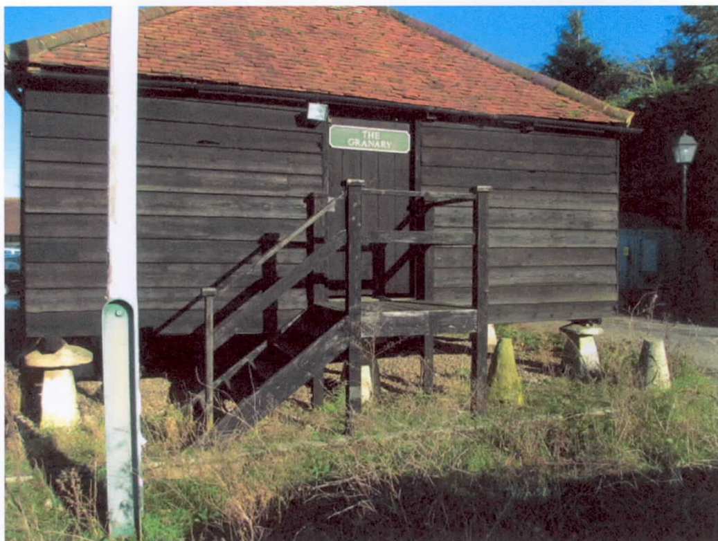
Fig 6: View of the Granary
