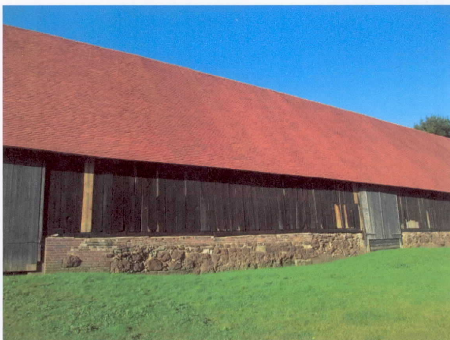
Fig10: Eastern elevation of the Great Barn owned by English Heritage
