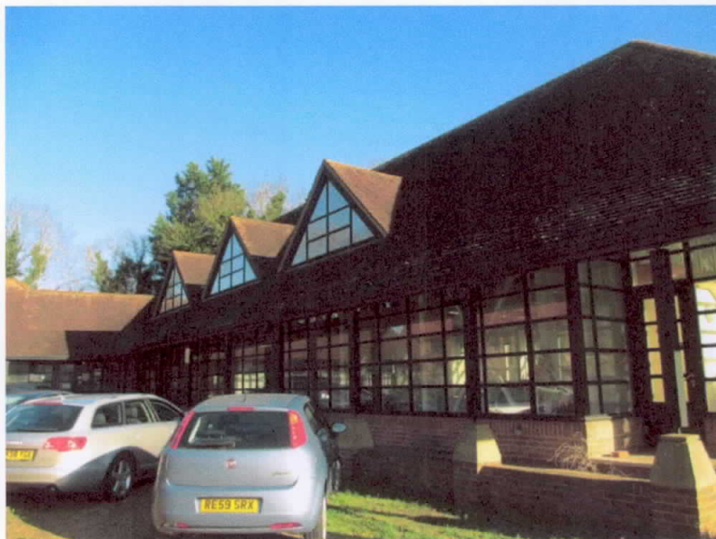
Fig 7: View of the Office Barn
