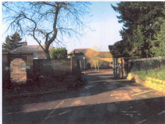
Fig 15: The entrance to Manor Court
