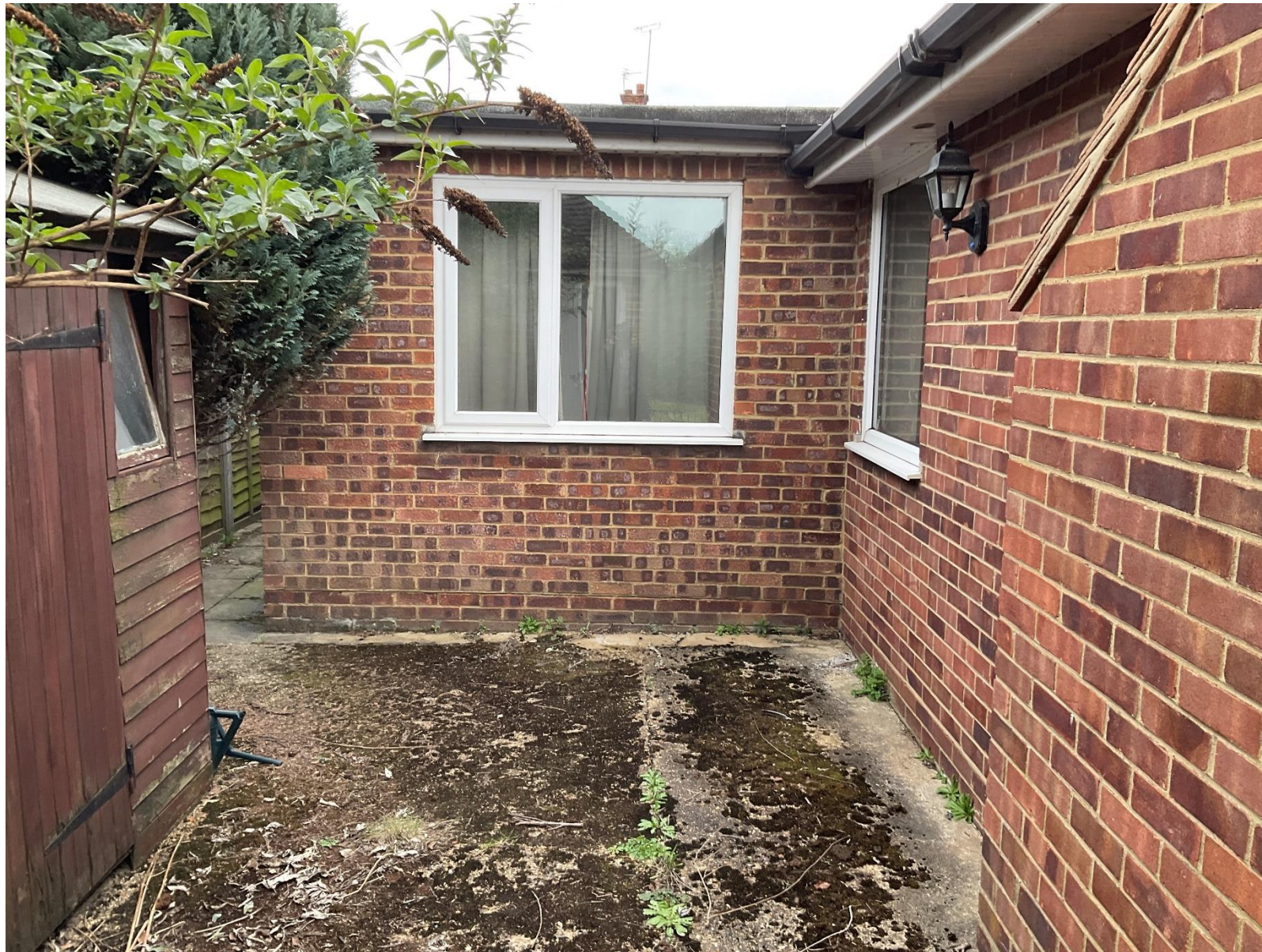
SITE PHOTOS: 2, Mills Close, Uxbridge, UB10 0JY
