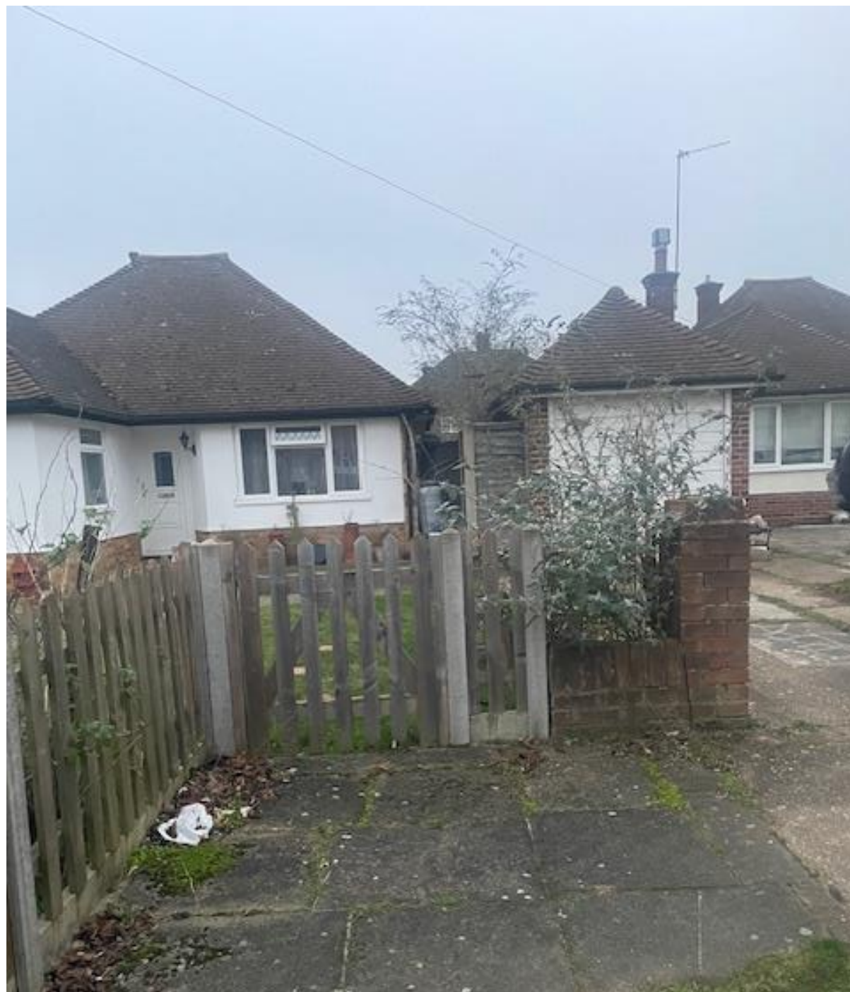
SITE PHOTOS: 2, Mills Close, Uxbridge, UB10 0JY
