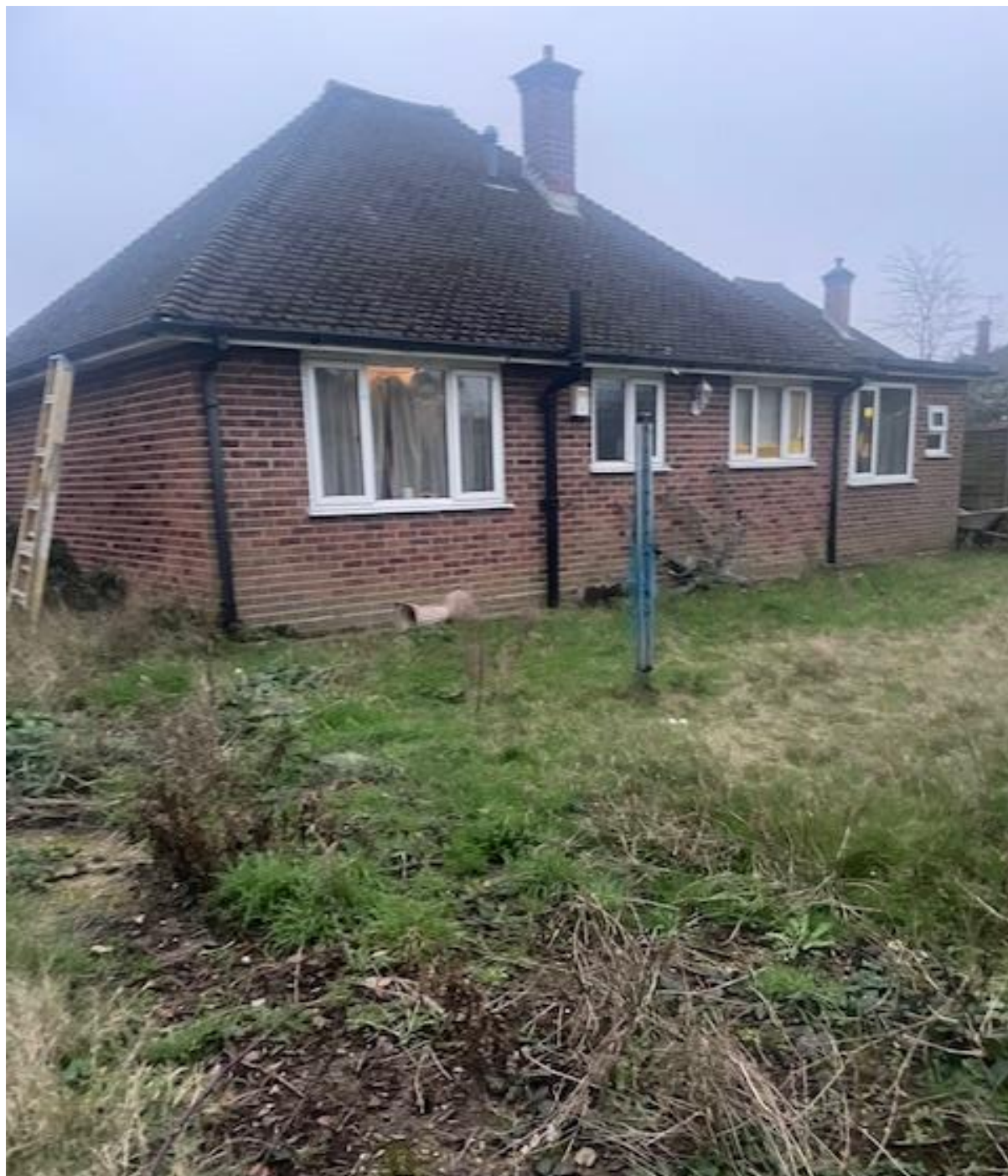
SITE PHOTOS: 2, Mills Close, Uxbridge, UB10 0JY
