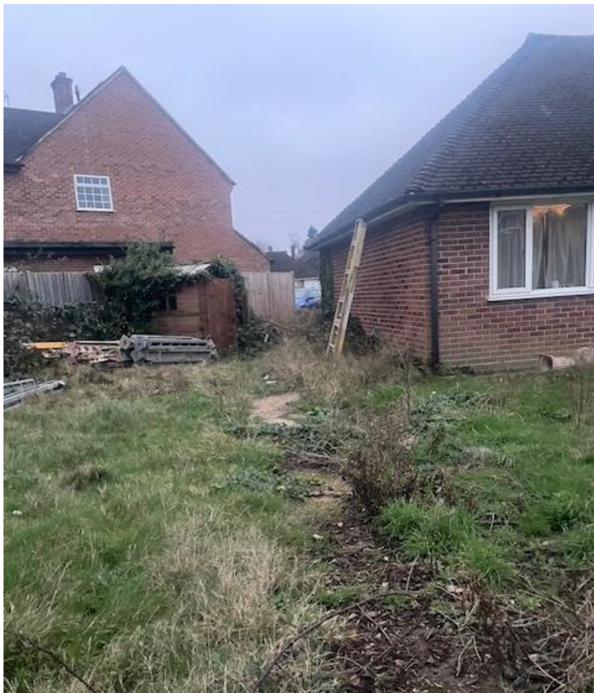
SITE PHOTOS: 2, Mills Close, Uxbridge, UB10 0JY
