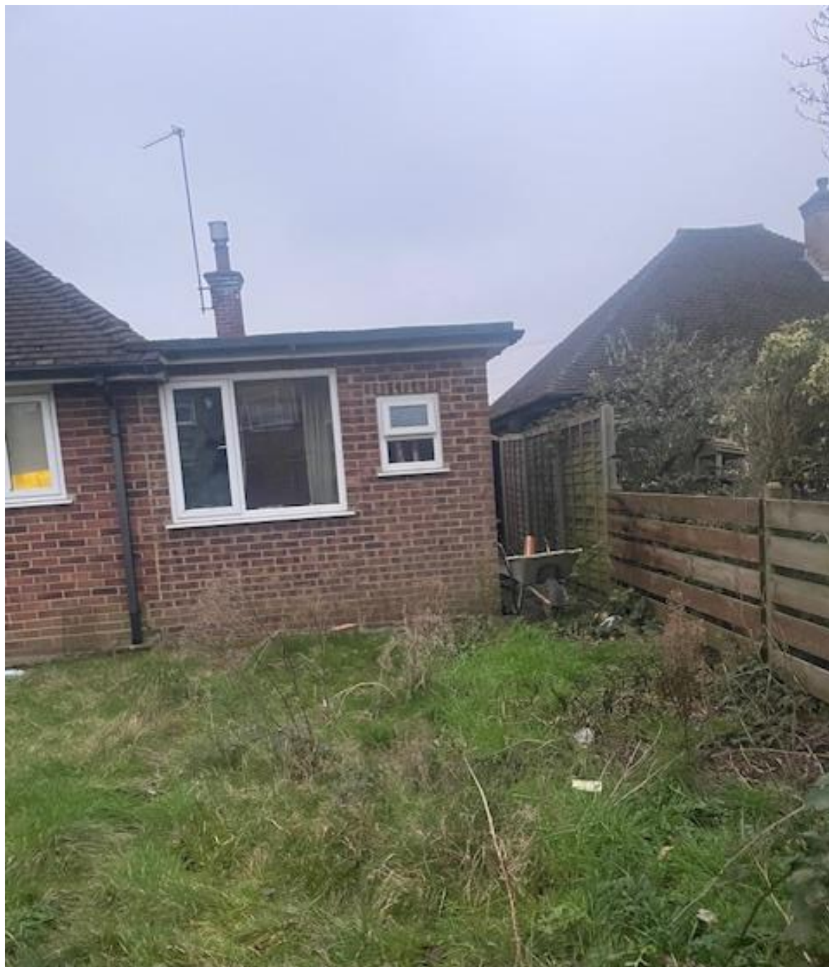
SITE PHOTOS: 2, Mills Close, Uxbridge, UB10 0JY
