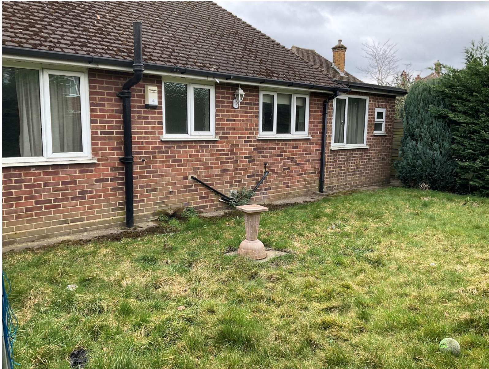
SITE PHOTOS: 2, Mills Close, Uxbridge, UB10 0JY
