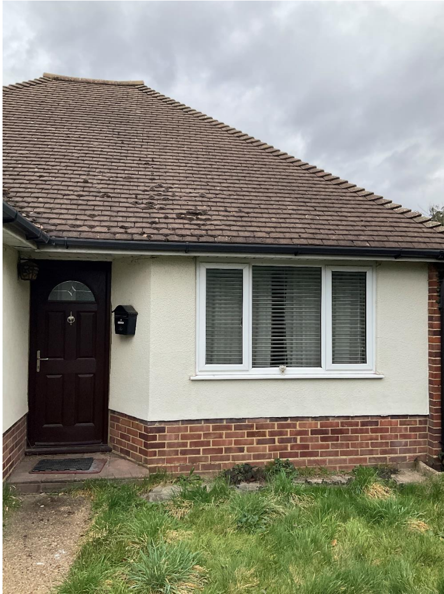
SITE PHOTOS: 2, Mills Close, Uxbridge, UB10 0JY
