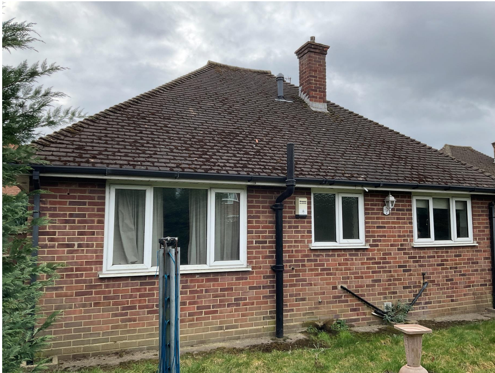
SITE PHOTOS: 2, Mills Close, Uxbridge, UB10 0JY
