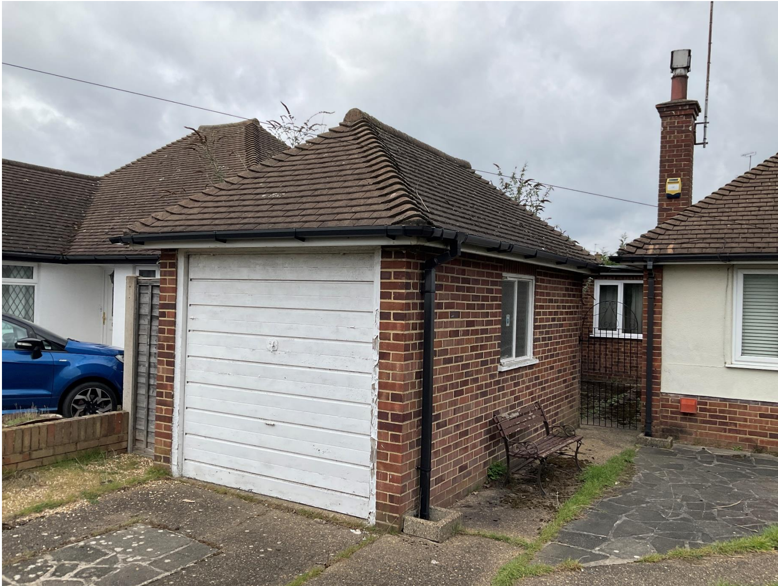
SITE PHOTOS: 2, Mills Close, Uxbridge, UB10 0JY
