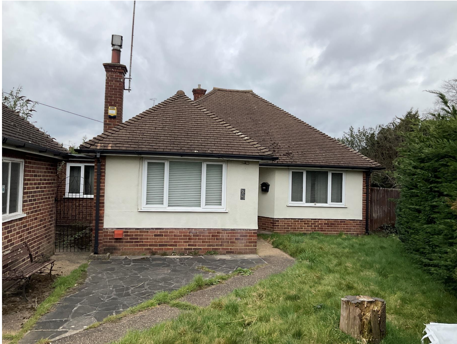
SITE PHOTOS: 2, Mills Close, Uxbridge, UB10 0JY
