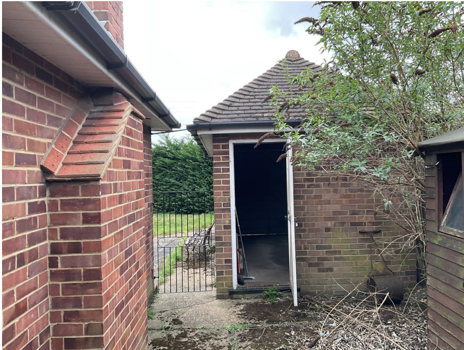
SITE PHOTOS: 2, Mills Close, Uxbridge, UB10 0JY
