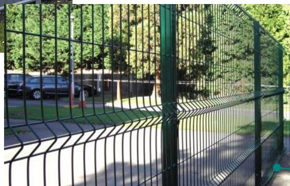
Proposed 2.2m visually secure fencing on the outer face of MUGA
